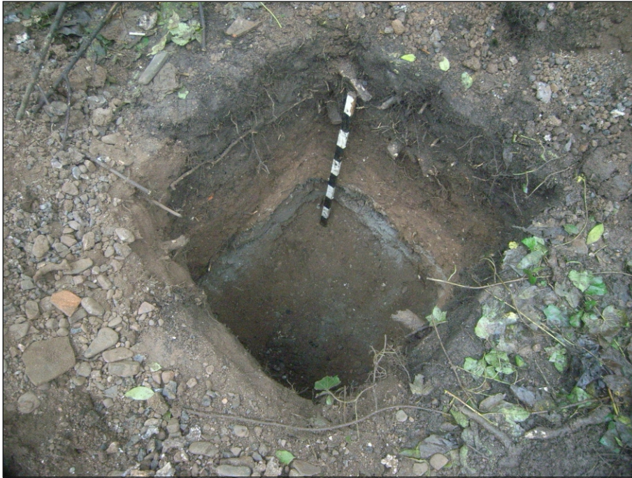
Zone 6 – Northbrook and existing Woodland Test Pit 16 demolition rubble to 1.20m from the south
