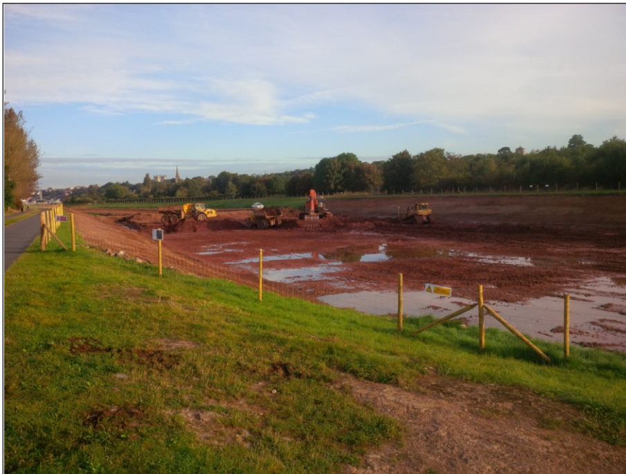
Plate 6: Watching brief area showing excavation methodology, viewed from the south
