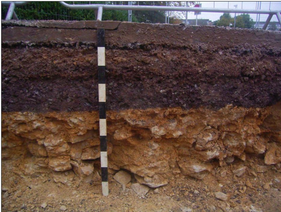
Plate 2: Representative section showing made ground from the South
