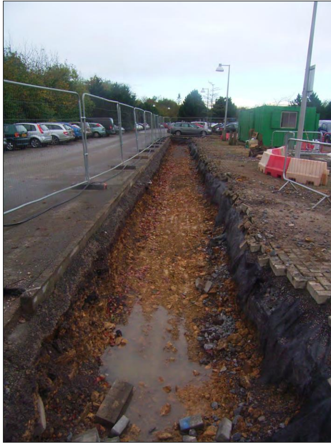
Plate 1: Service diversion trench from the East
