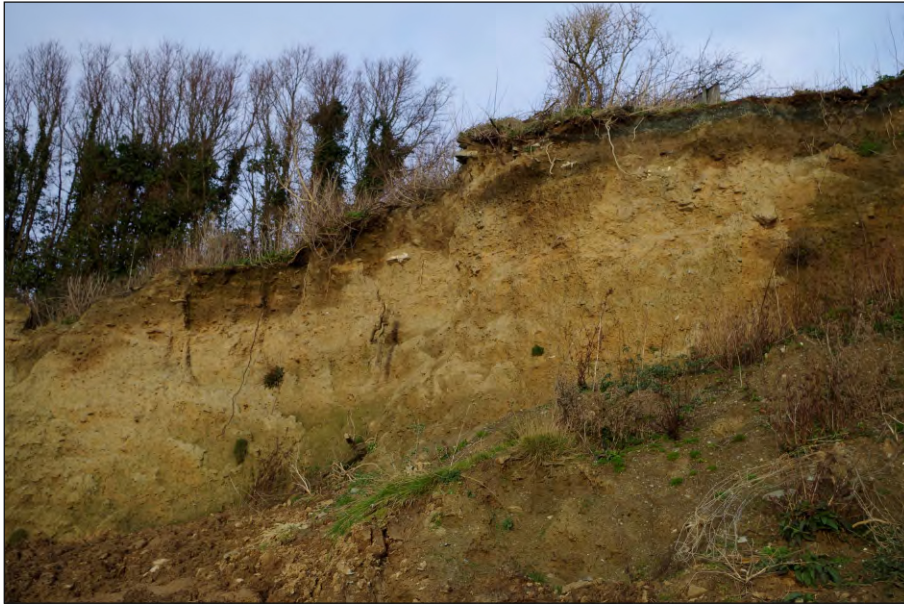
Plate 5: View of collapsed cliff-top from the South
