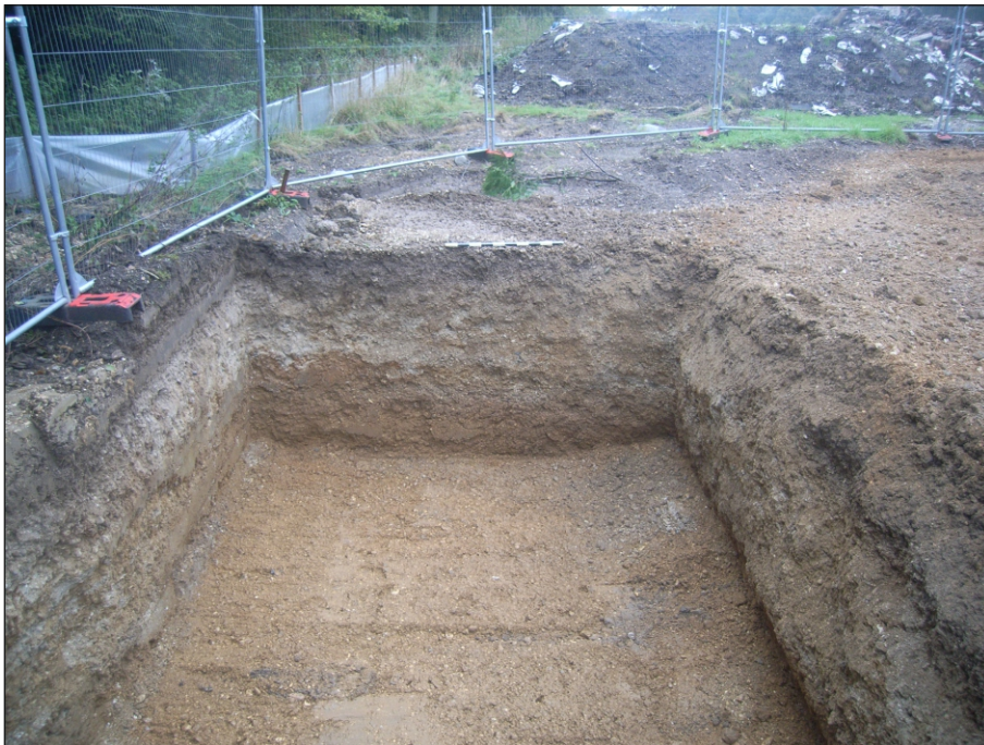
Plate 2: Stratigraphy revealed in water sump excavation
