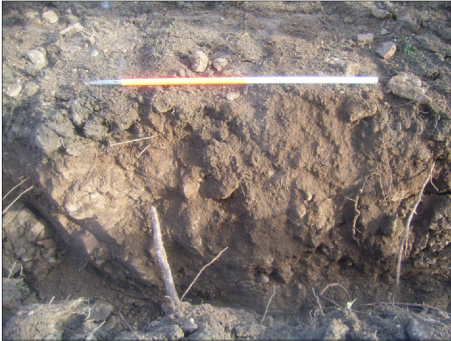
Plate 1: Southwest facing shot of Trench 1
