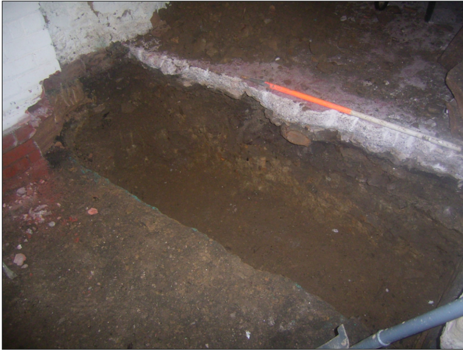
Plate 5: General view of Trench 2 , looking northwest
