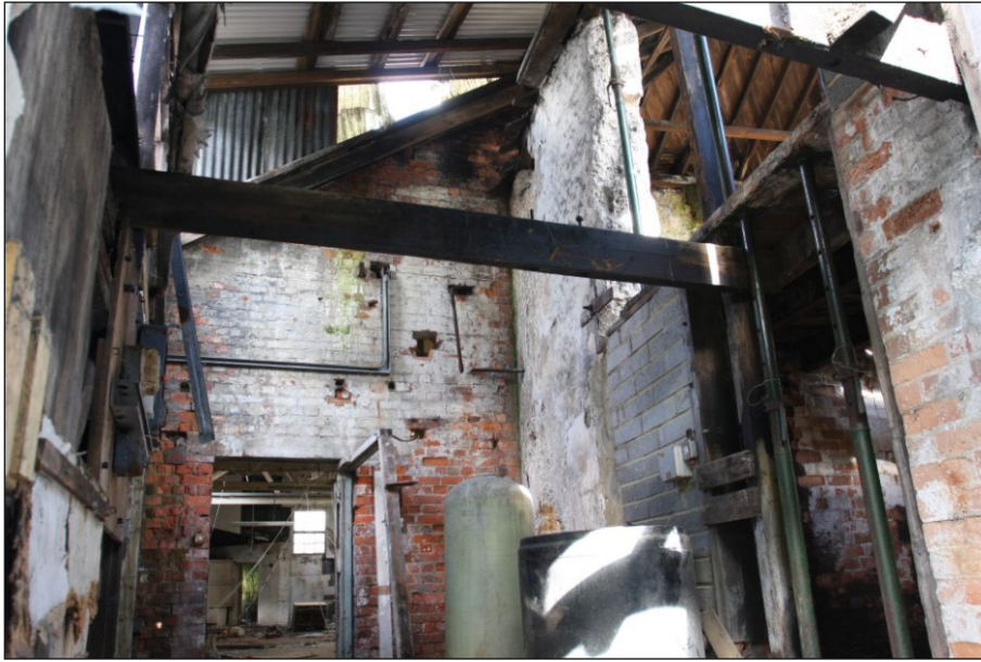
Plate 7: Building 2 interior viewed from the south-east
