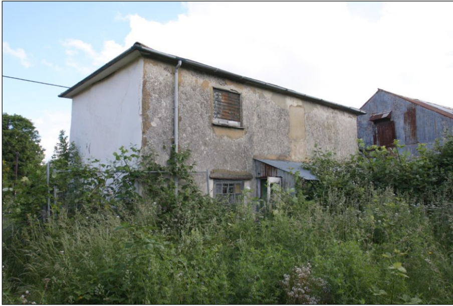
Plate 21: Building 5 viewed from the south-west
