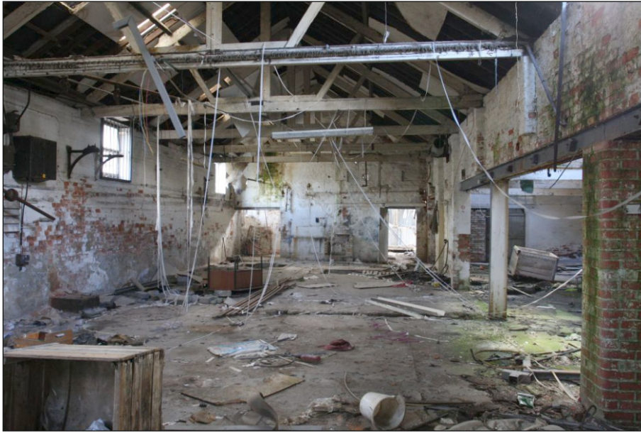
Plate 9: Building 3 interior viewed from the west
