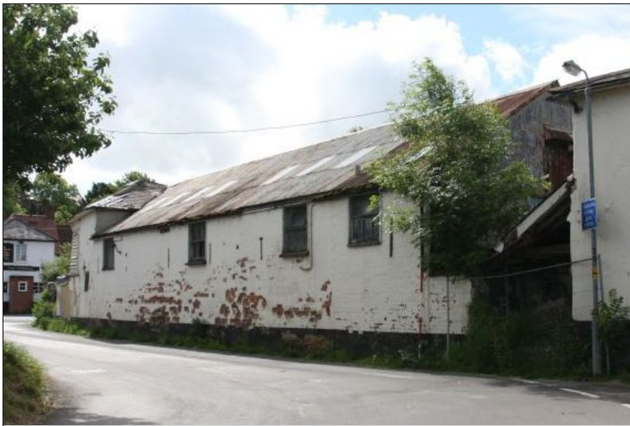
Plate 8: Building 3 north elevation viewed from the north-west
