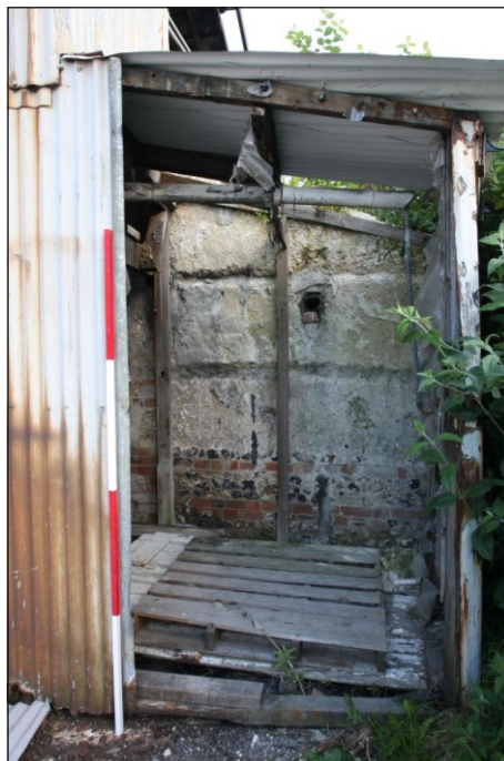
Plate 6: Building 2 south-east corner entrance
