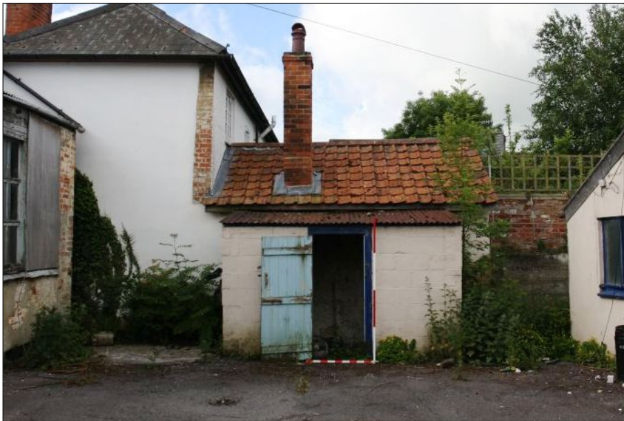
Plate 26: Building 7 north elevation
