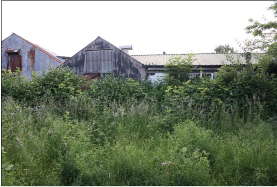
Plate 15: Building 4 west elevation. Building 3 is to the left
