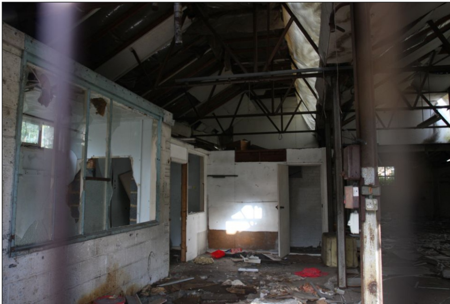
Plate 18: Building 4 interior of the south block viewed from the east
