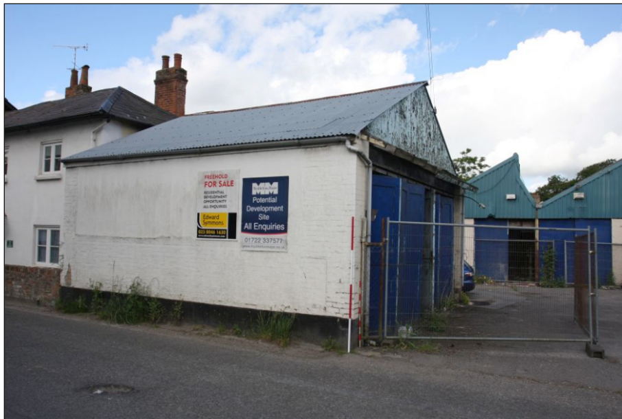
Plate 24: Building 6 viewed from the north-east
