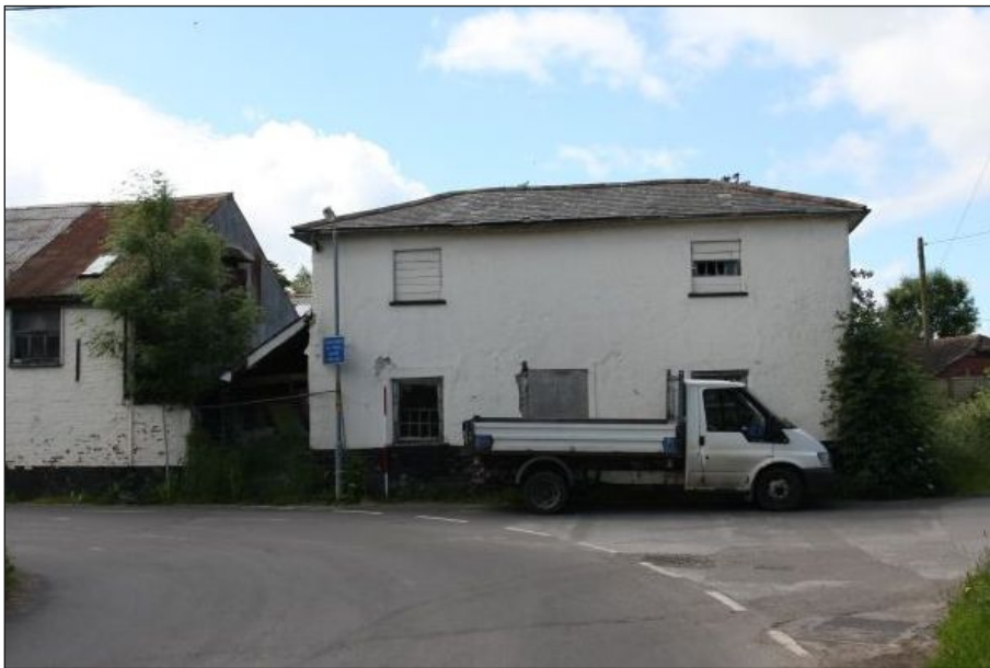
Plate 20: Building 5 north elevation
