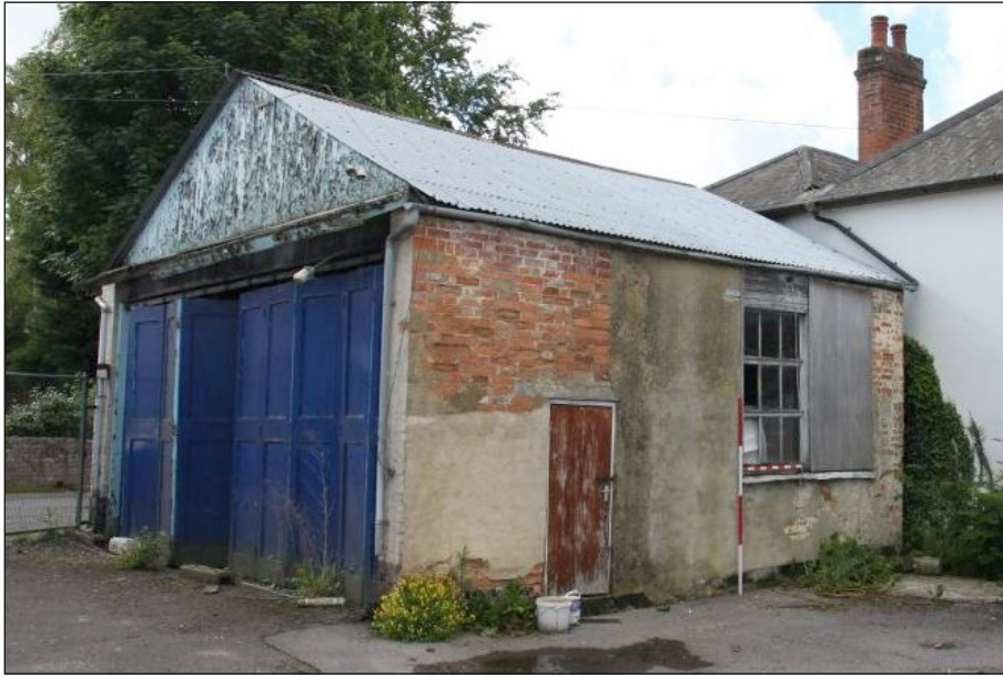
Plate 25: Building 6 viewed from the north-west
