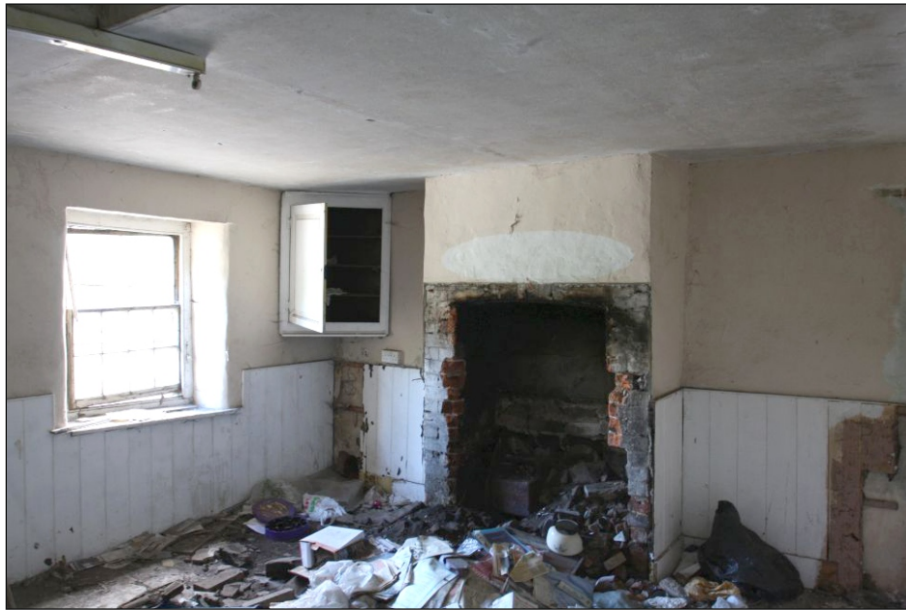
Plate 23: Building 5 ground floor east room, viewed from the south-west
