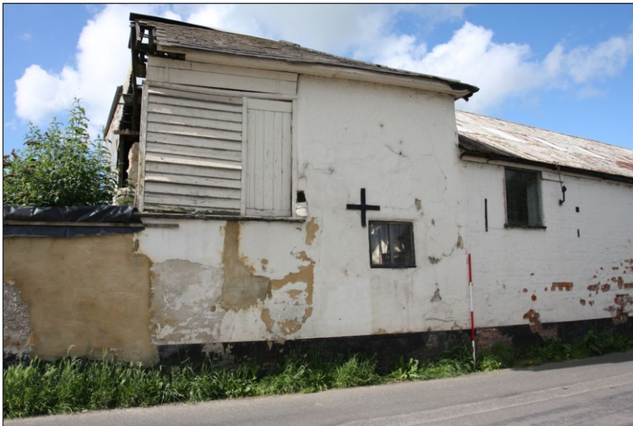
Plate 4: Building 2 north elevation
