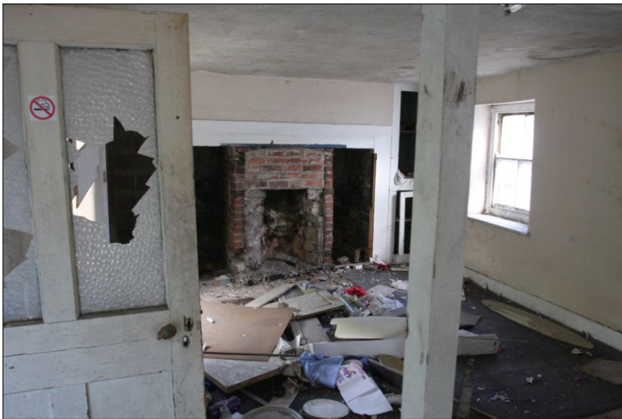
Plate 22: Building 5 ground floor west room, viewed from the south-east
