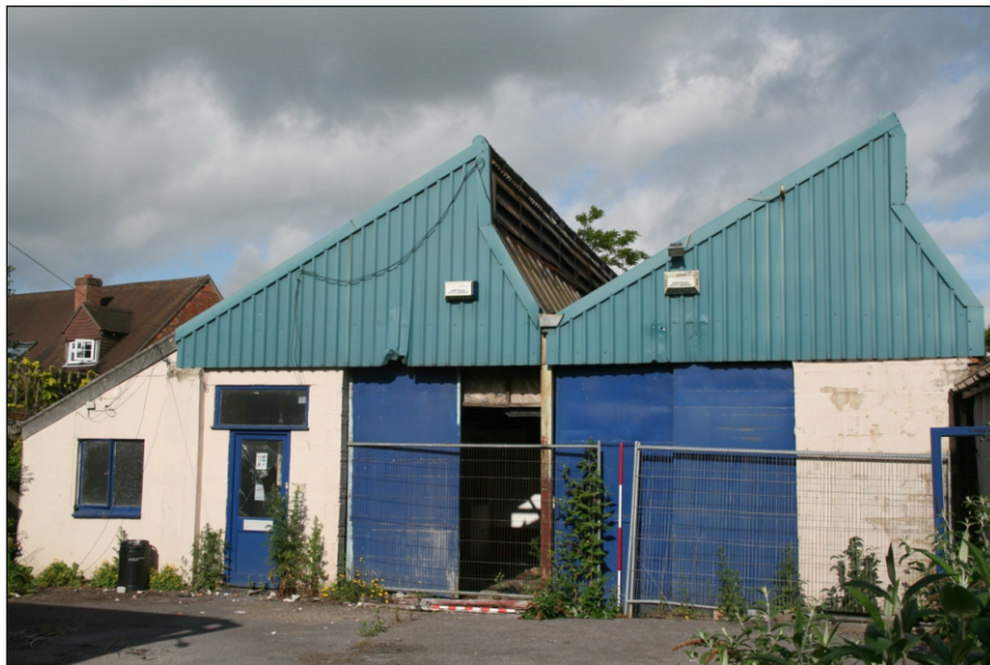
Plate 12: Building 4 south end of the east elevation
