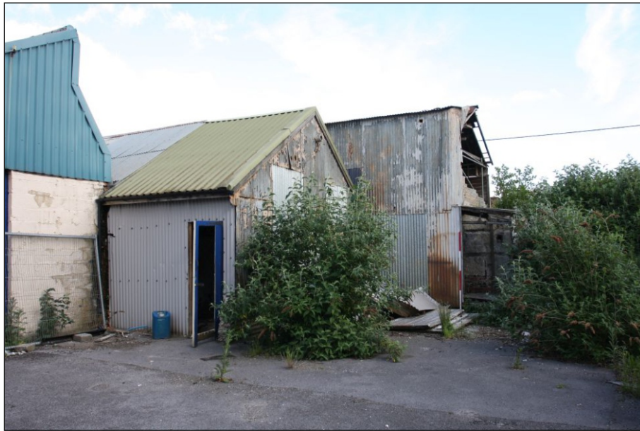
Plate 13: Building 4 north-east block. Building 2 is in the background
