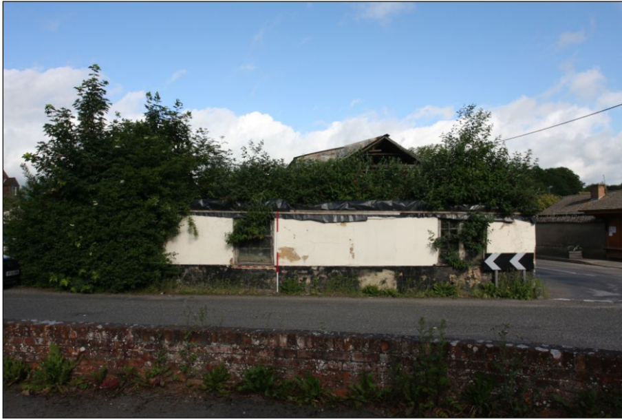
Plate 1: Building 1 east elevation
