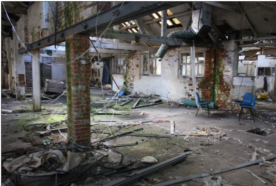
Plate 16: Building 4 interior of the north block viewed from the north-west
