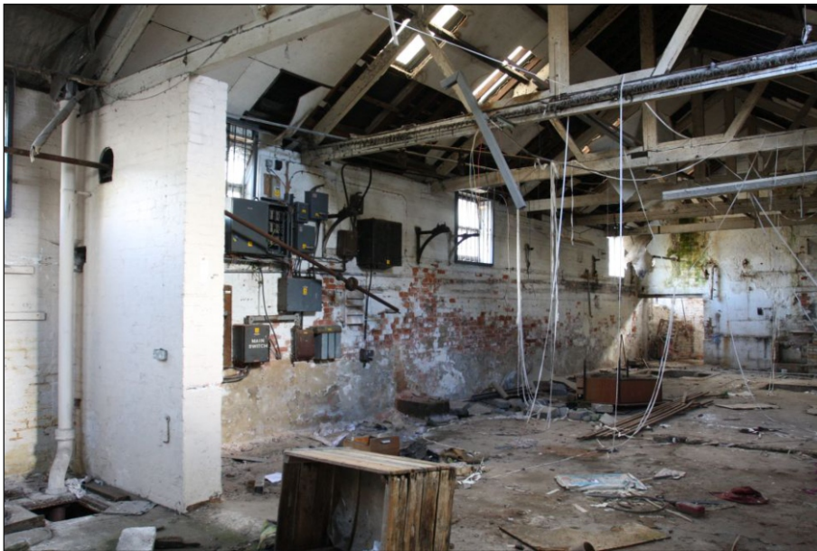
Plate 10: Building 3 interior north wall. Brackets for laundry machinery are still in-situ
