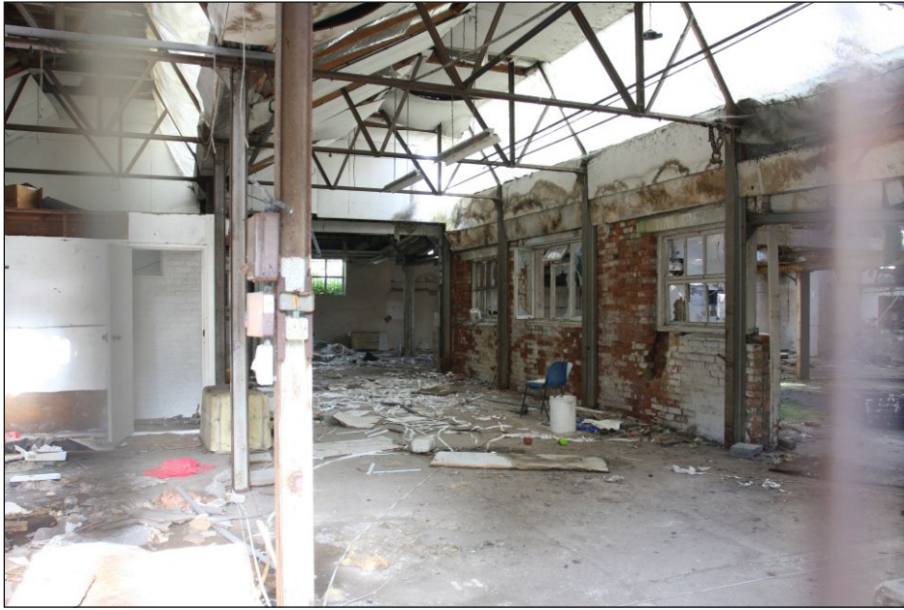
Plate 19: Building 4 interior of the central block viewed from the south-east
