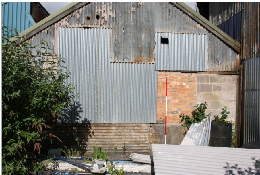
Plate 14: Building 4 east elevation of the north-east corner block
