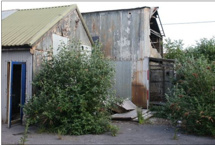
Plate 5: Building 2 south elevation partly obscured by Building 4 in left foreground
