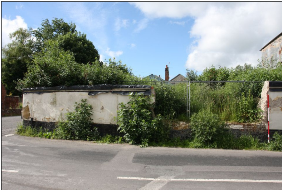
Plate 2: Building 1 east end of the north elevation
