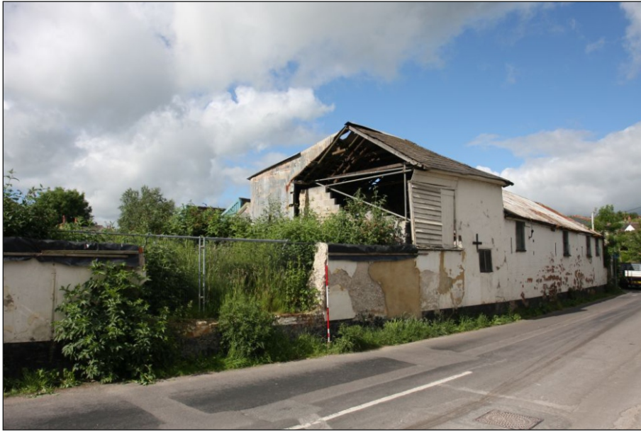
Plate 3: Building 1 north elevation and adjacent structures Buildings 2 and 3
