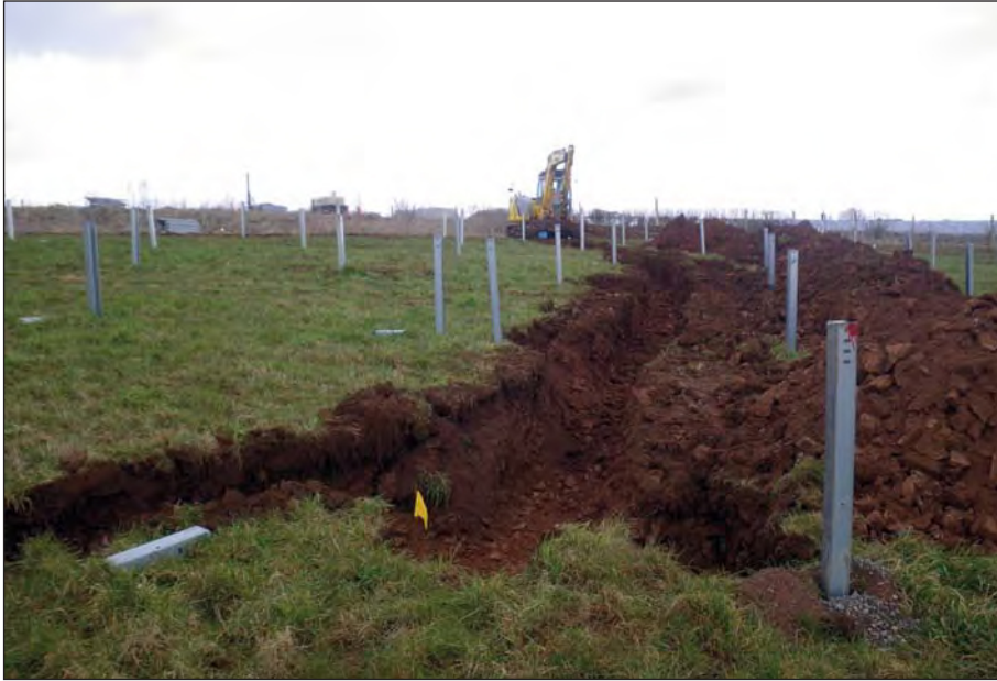
Plate 1: Overall view of Trench 2 from the south
