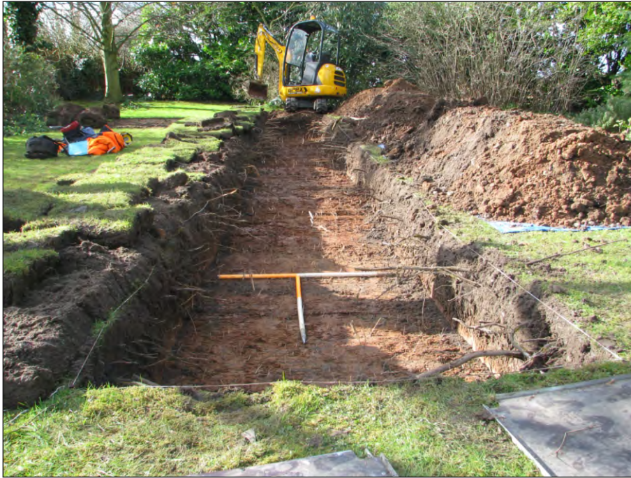
Plate 1: General shot of Trench 8
