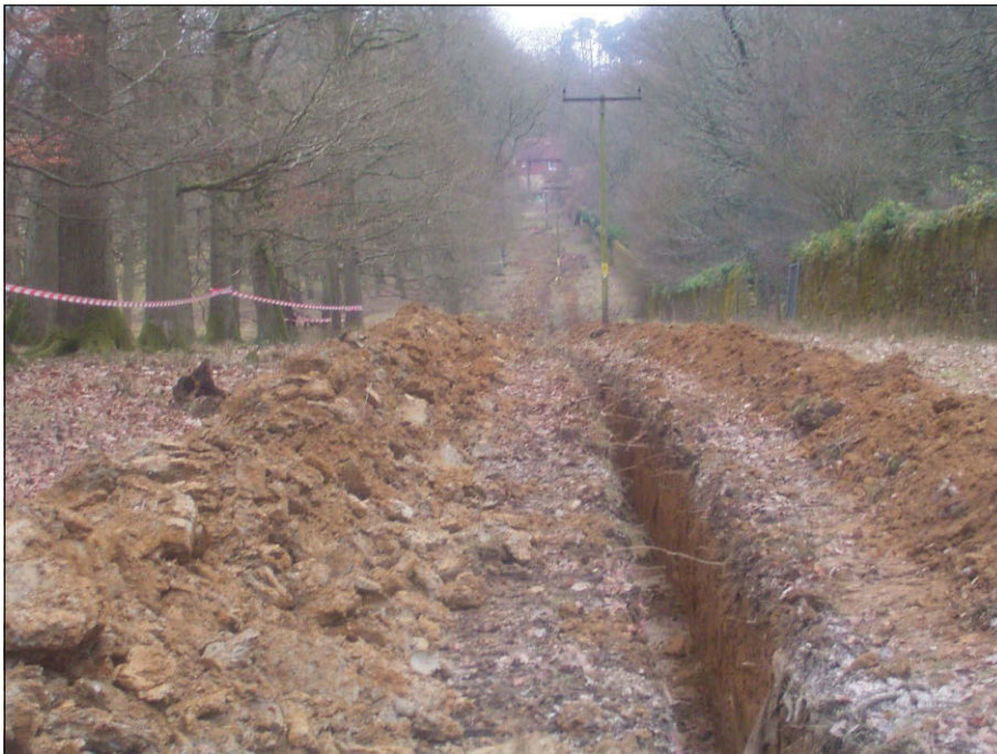
Plate 5: Cable trench from the east
