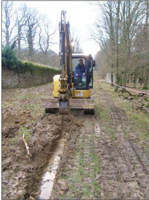
Plate 6: Working shot illustrating wet conditions
