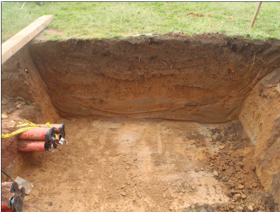
Plate 4: Trench 6 from north
