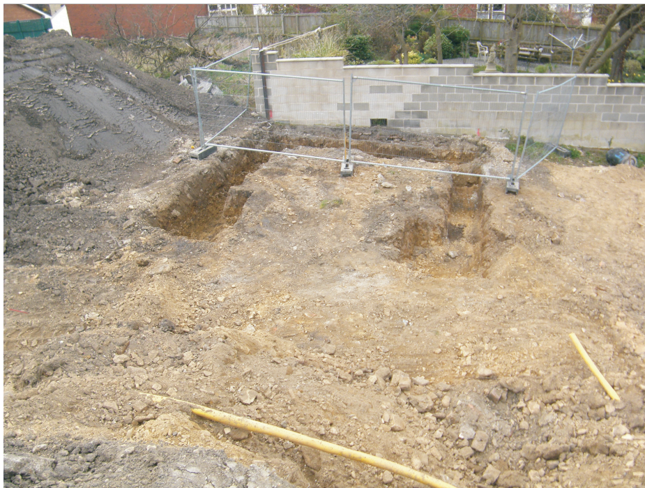
Plate 2: Excavated garage foundation trench, looking north-west
