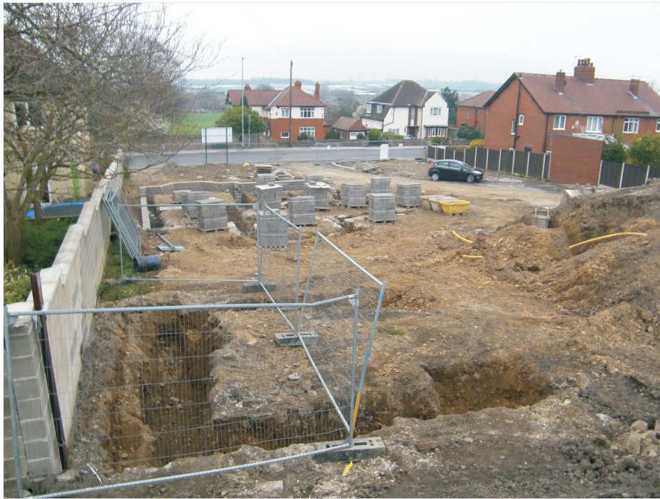
Plate 1: General view of foundation trenches, looking north-east
