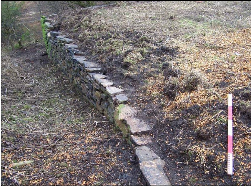
Plate 23 – General view along western wall of platform in Area G
