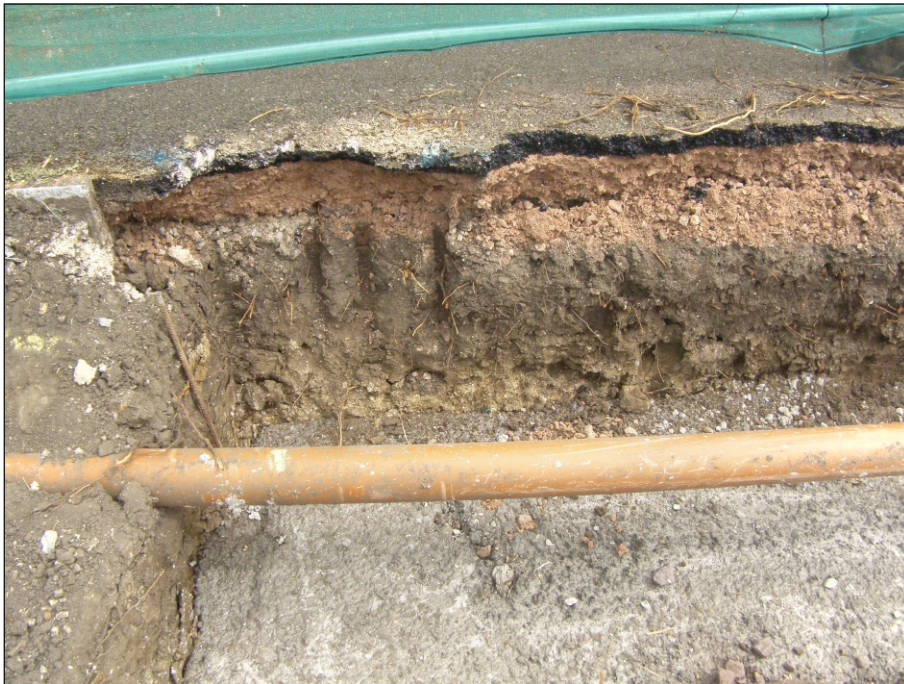
Plate 3: Sample section, with concrete foundations
