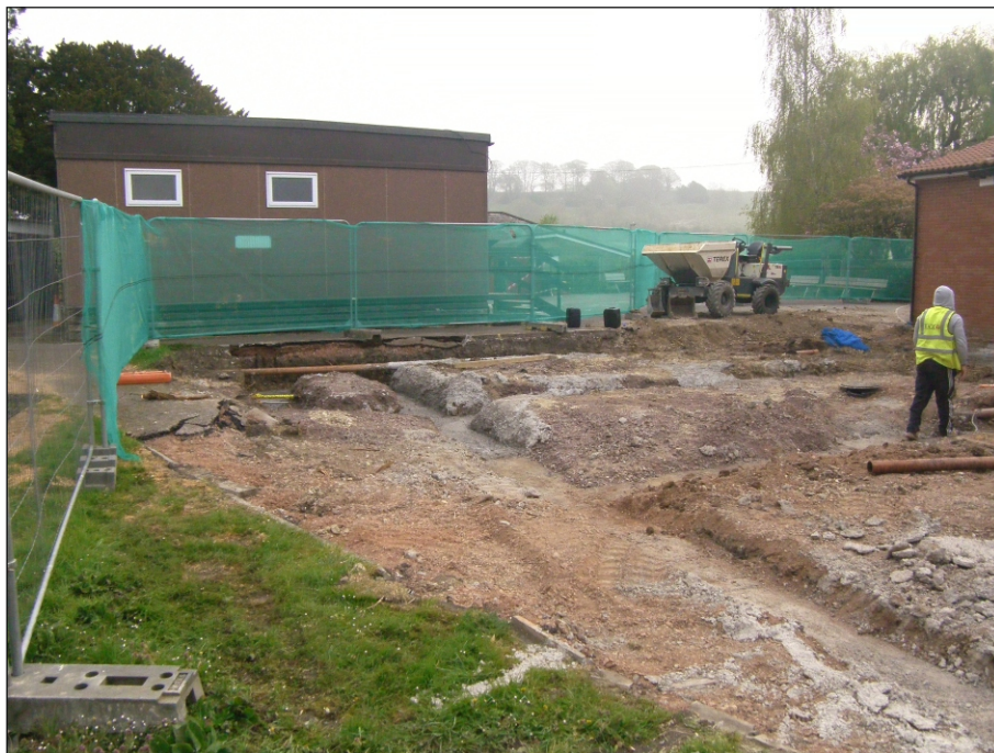
Plate 2: General site shot, from the south
