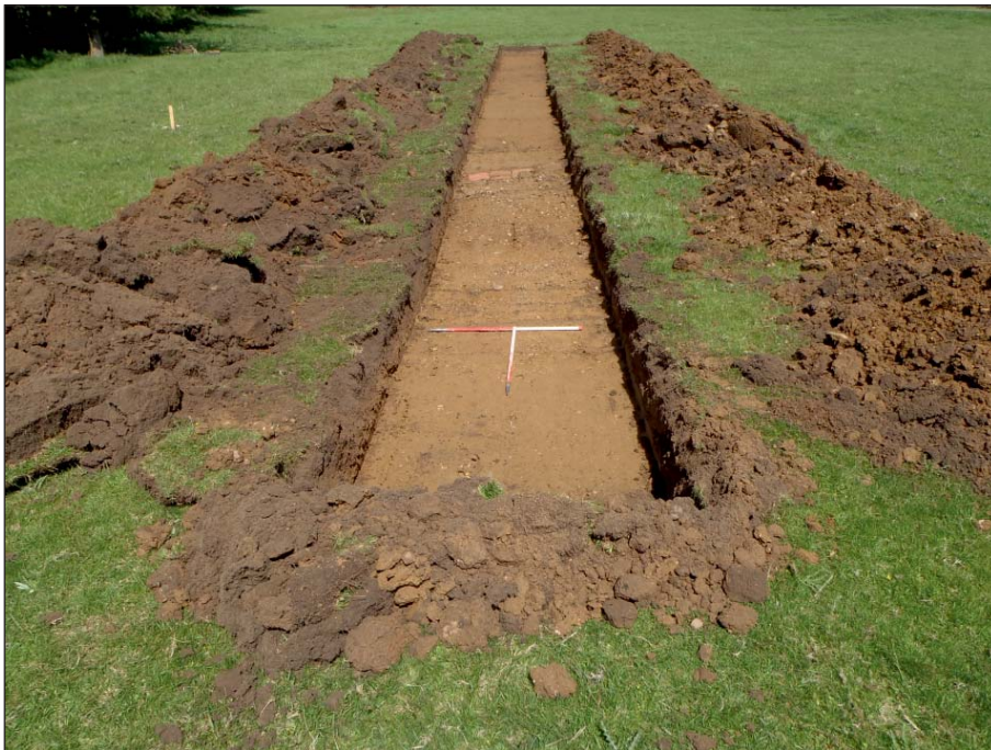
Plate 4: Trench 4 from southeast
