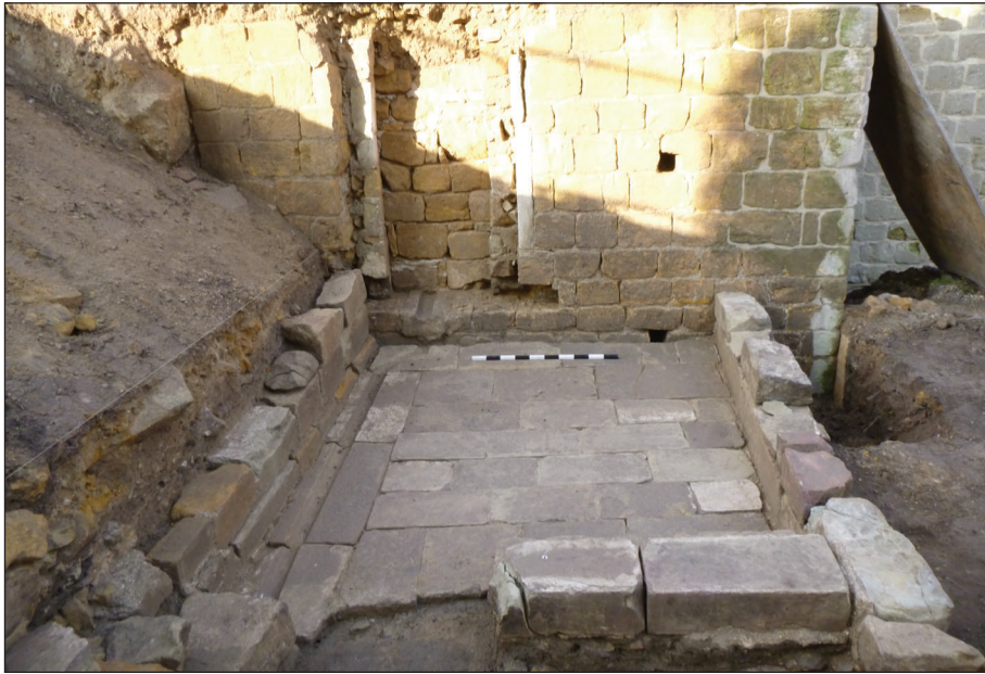
Plate 7: The northern side of the Piper Tower, door 6506 and structure 6508
