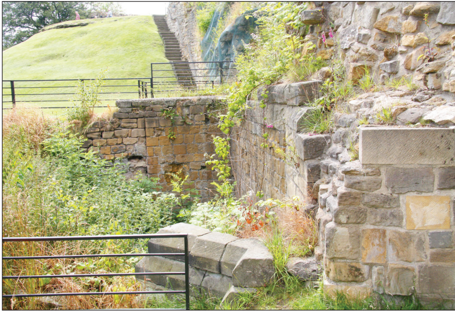
Plate 1: The Sallyport before excavation
