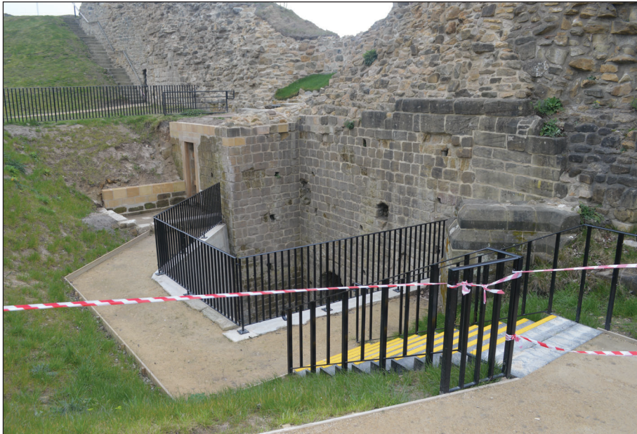
Plate 2: The Sallyport following conservation and installation of the new visitor access
