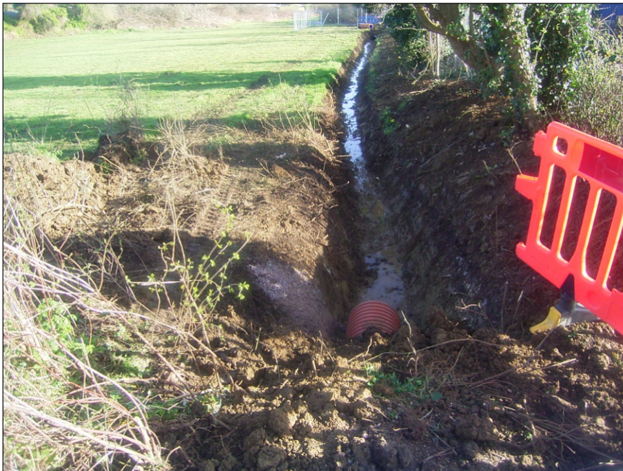
Plate 2: Southern section of drainage ditch in Long Close looking north
