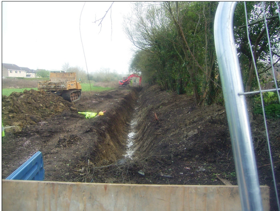
Plate 3: Northern section of drainage ditch in Long Close looking north
