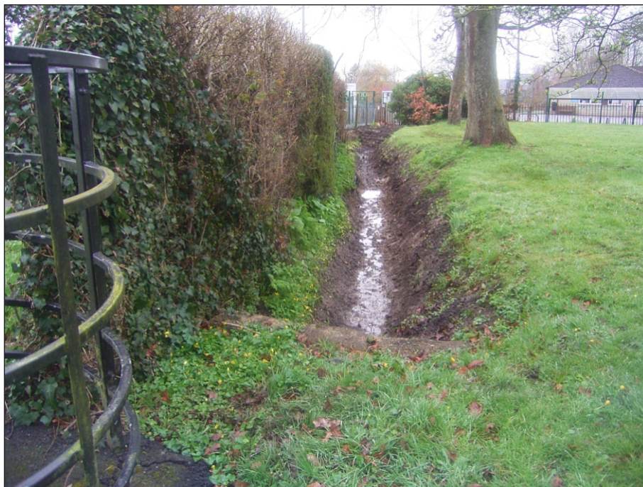
Plate 4: Section of drainage ditch in cemetery boundary looking east
