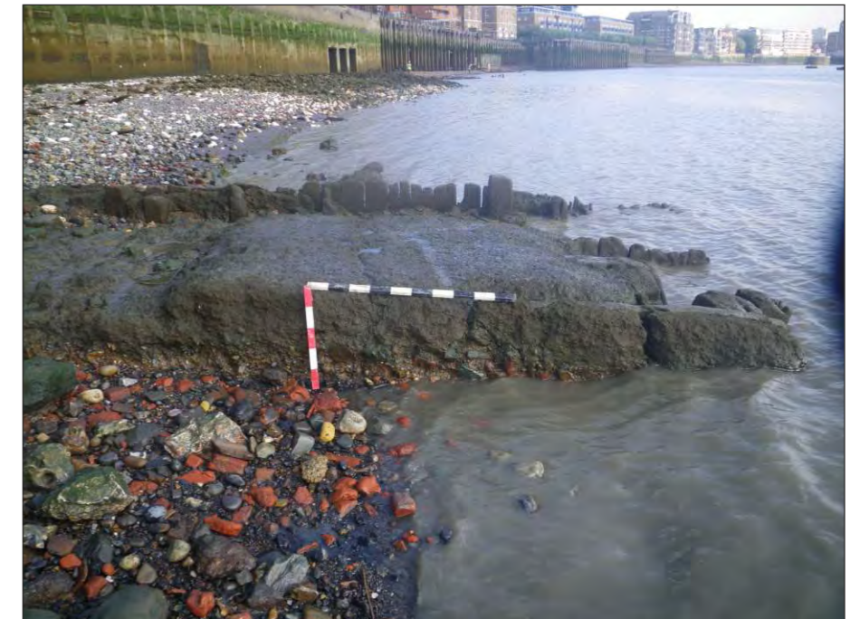
Plate 14: View from south-west of structure 9007 showing depth of concrete
