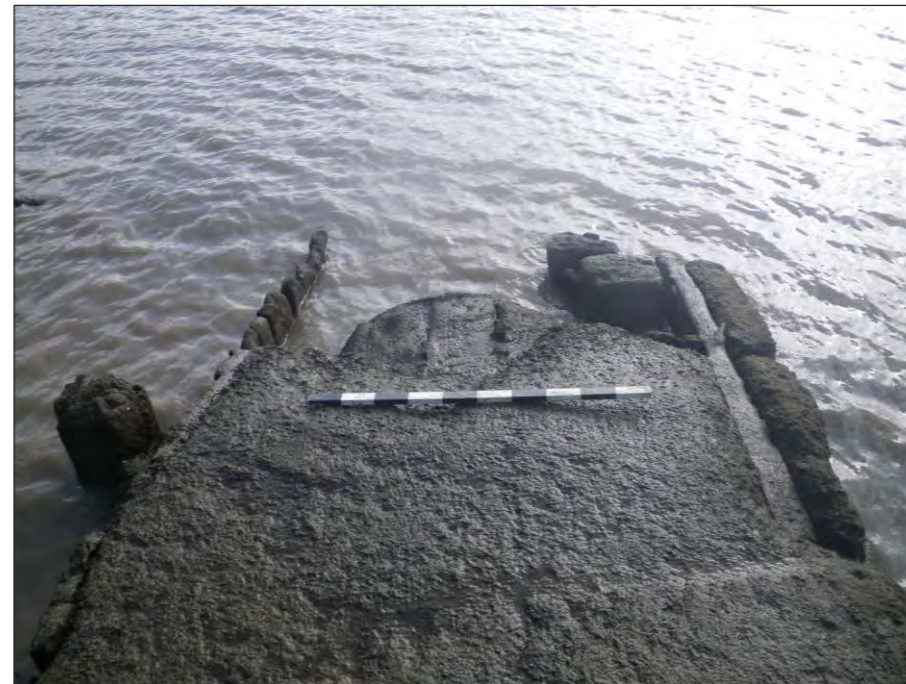
Plate 13: View from north-west showing detail of south-western part of structure 9007 with concrete infilling and timber covering outlet underneath
