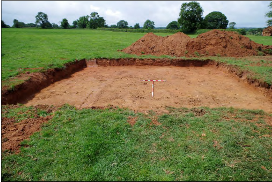
Plate 1: Excavation area, looking west
