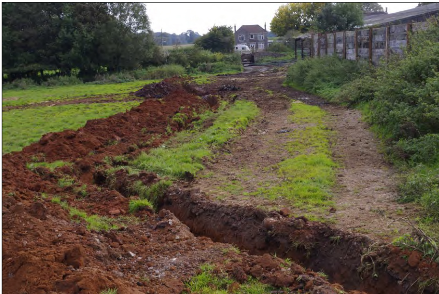
Plate 2: Cable trench to the north of Knitts Farm, looking south-east
