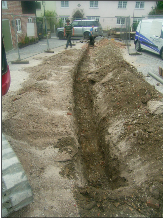
Plate 3: View of excavated pipe trench, from east
