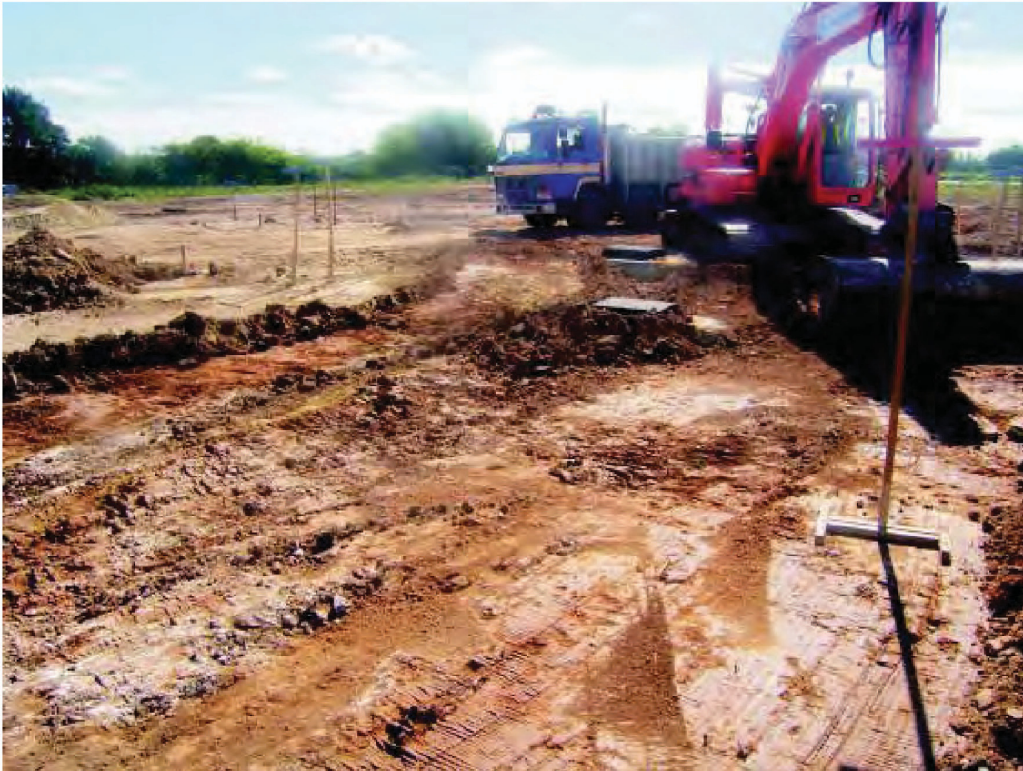
Plate 2. Phase 2 - Roadway stripping
