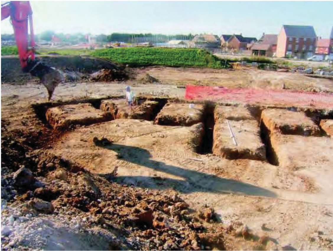
Plate 3. Phase 3 - Footing excavations
