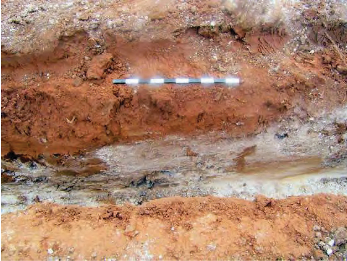
Plate 1. Phase 1 - Drainage trench from East
