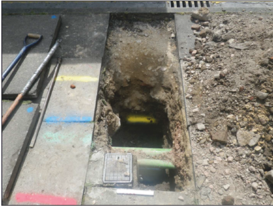
Plate 1: Trial hole 27, camera facing north-east
