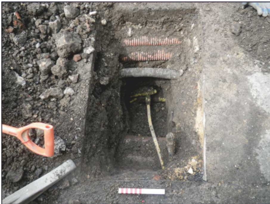
Plate 2: Trial hole 39, camera facing north
