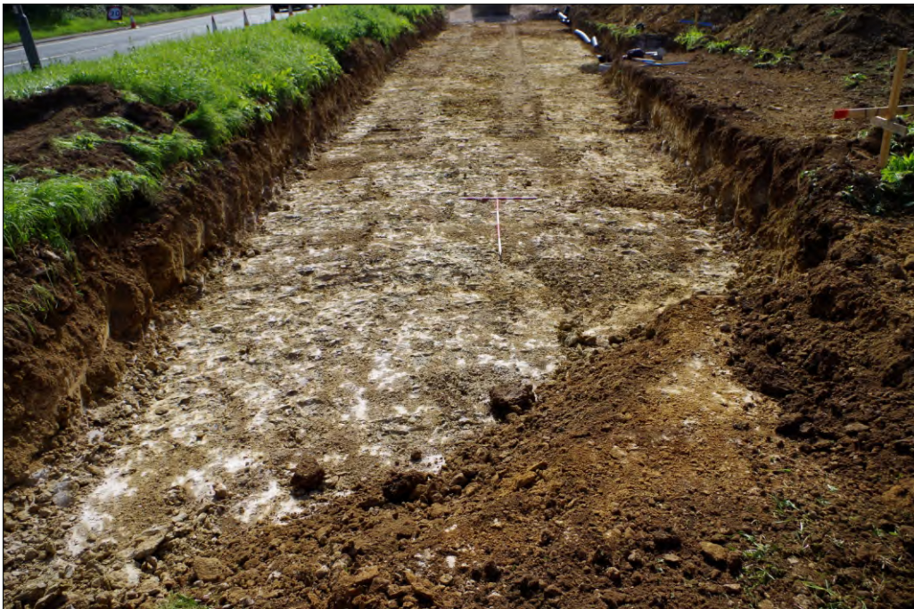
Plate 4: Ground reduction to the north of Brook Roundabout, looking south
