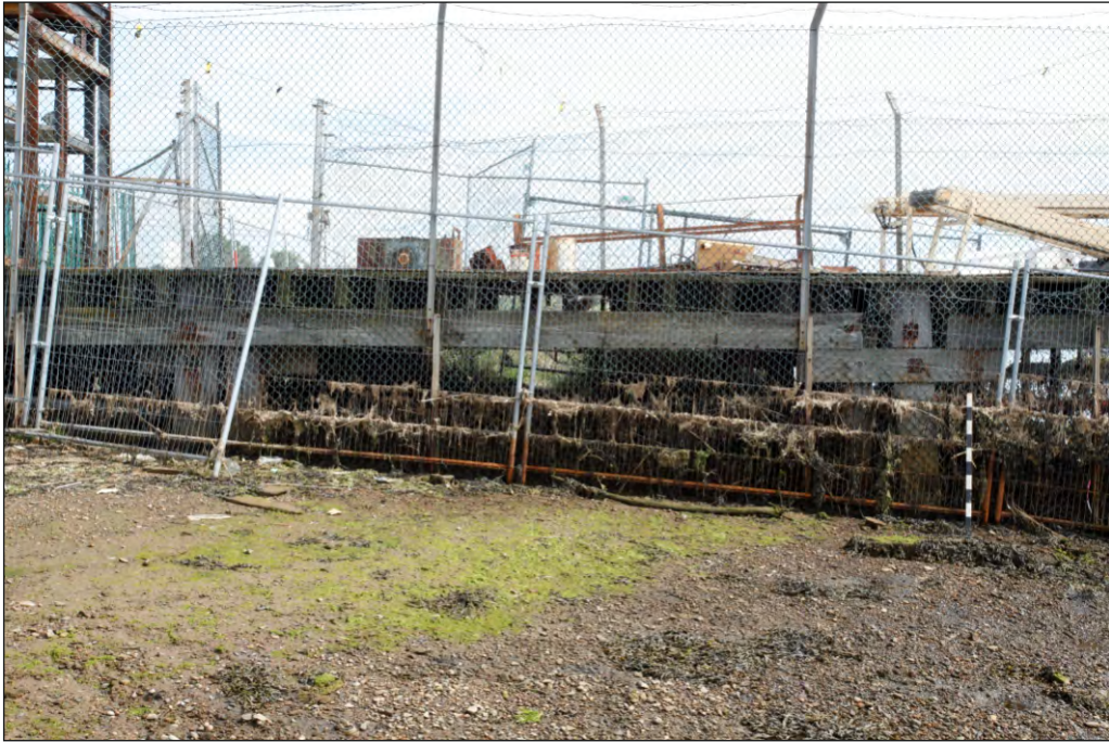
Plate 13: South-west elevation of the jetty showing recent replacement piles, looking north-east
