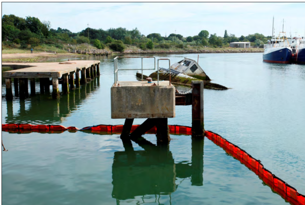
Plate 16: Detail of north-eastern mooring dolphin, looking north-east
