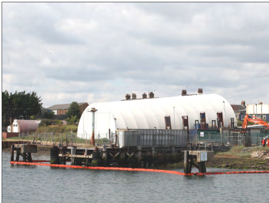
Plate 6: General view of the jetty and former Esso depot, looking west
