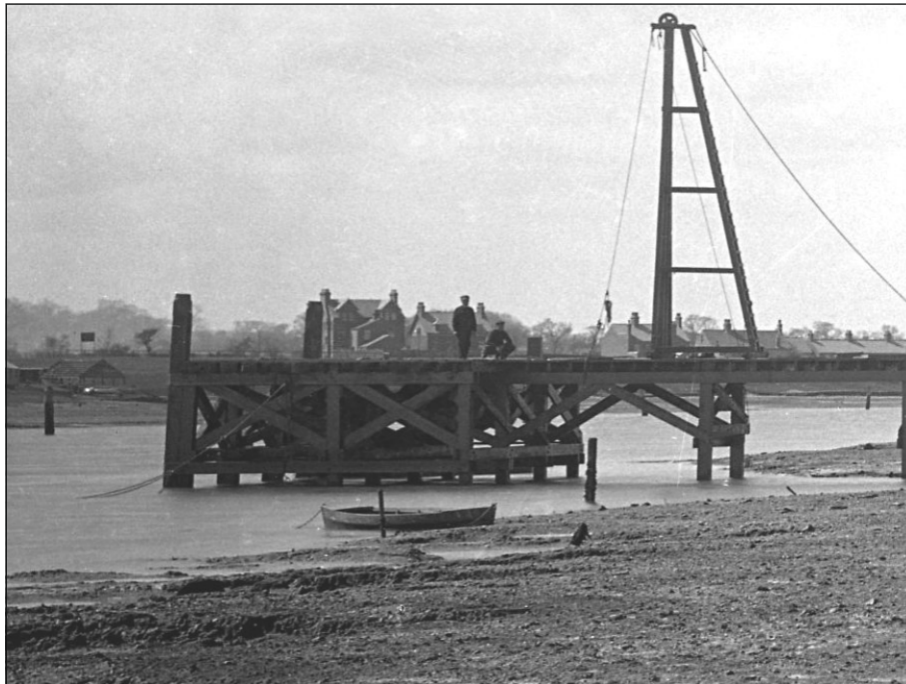
Plate 3: Detail of c 1901 photograph of the AAOC jetty, looking south-west, reproduced courtesy of Suffolk Records Office (SRO 715/A3/2/15)
