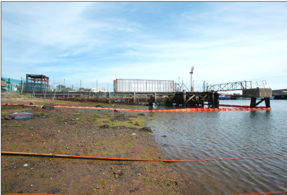
Plate 8: General view of the jetty, looking north-east
