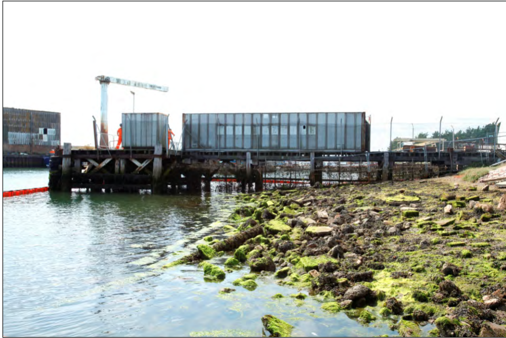
Plate 9: North-east elevation of the jetty, looking south-west
