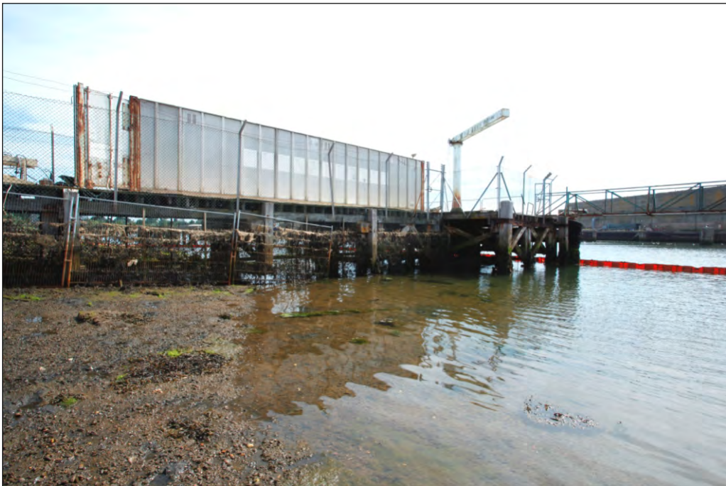
Plate 14: South-east elevation of the jetty, looking east
