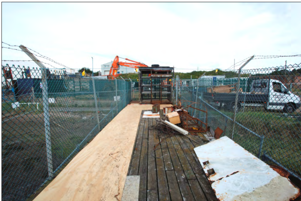
Plate 18: Deck of jetty, looking north-west
