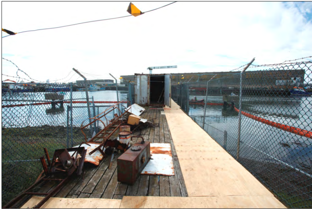
Plate 17: Deck of jetty, looking south-east
