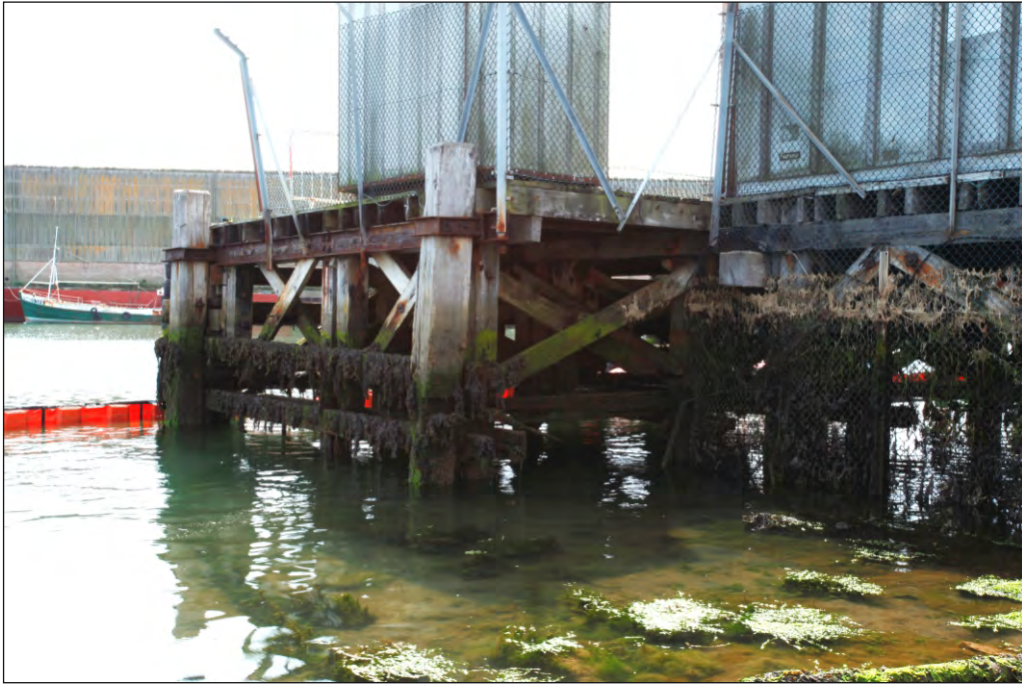
Plate 11: Detail of south-eastern end of the jetty (north-east side), looking south
