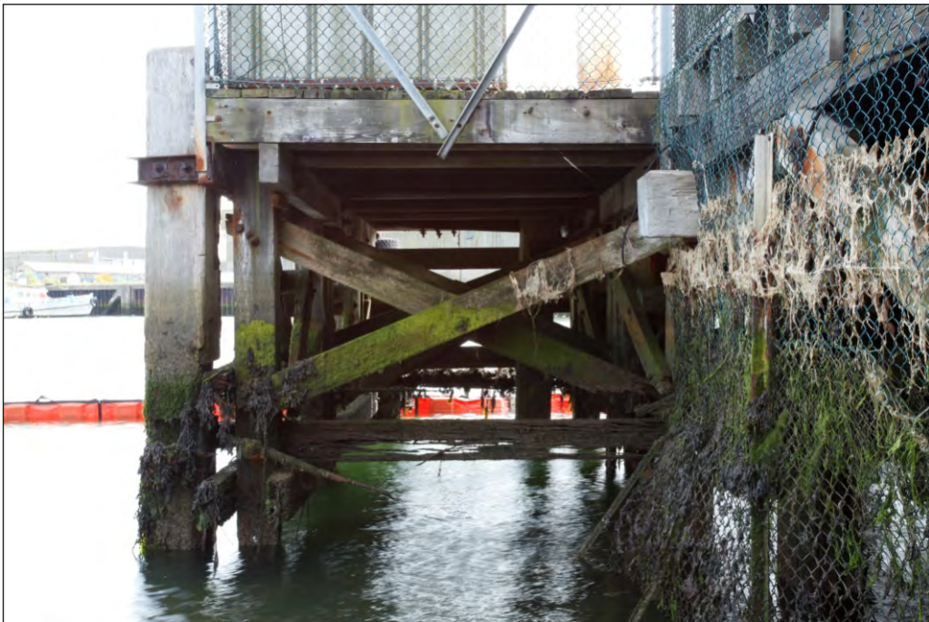
Plate 12: Detail of south-eastern end of the jetty (north-east side), looking south-east
