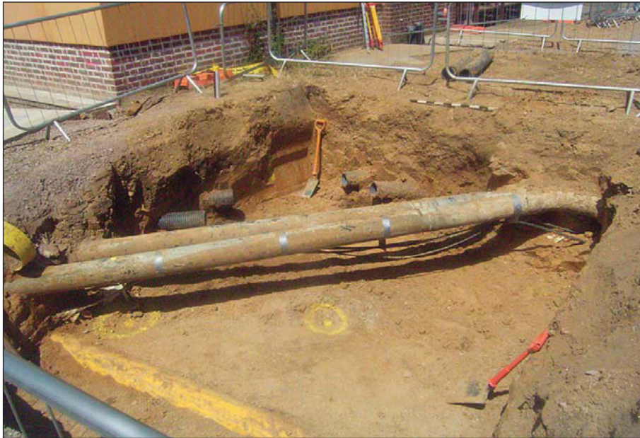
Plate 1: View of Trench 5 from the south-west showing utility services
