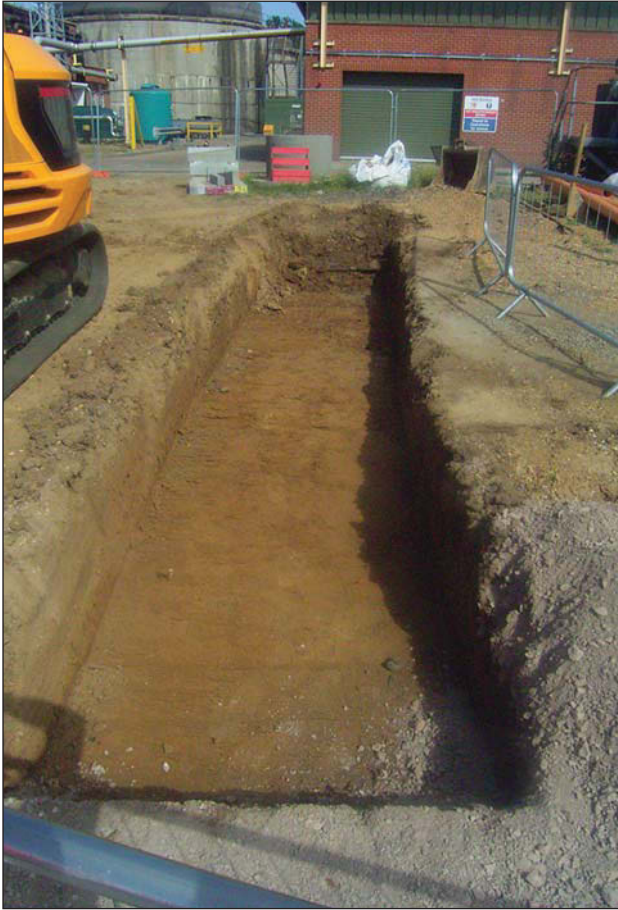
Plate 3: Trench 6 viewed from the west
