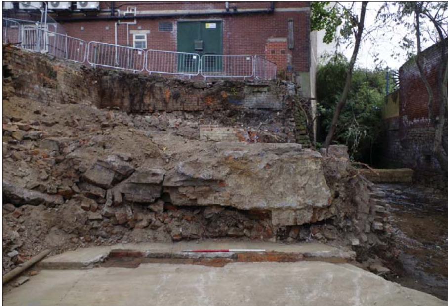
Plate 7: Foundation of redbrick wall 1007 from south
