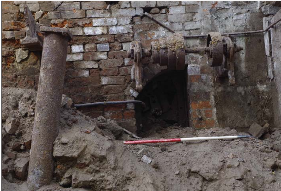
Plate 1: Steel girder and pier (1014) shown in left of shot from east
