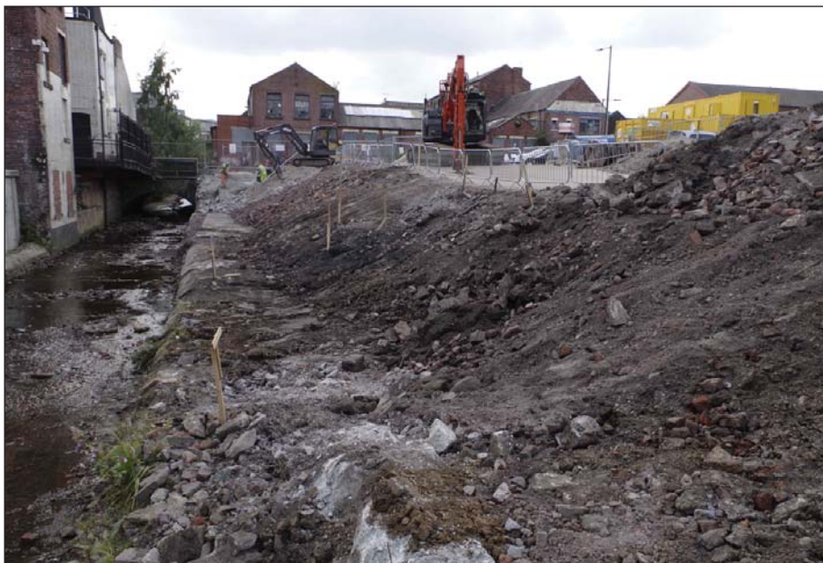
Plate 12: Negative result of watching brief along southern riverside from north
