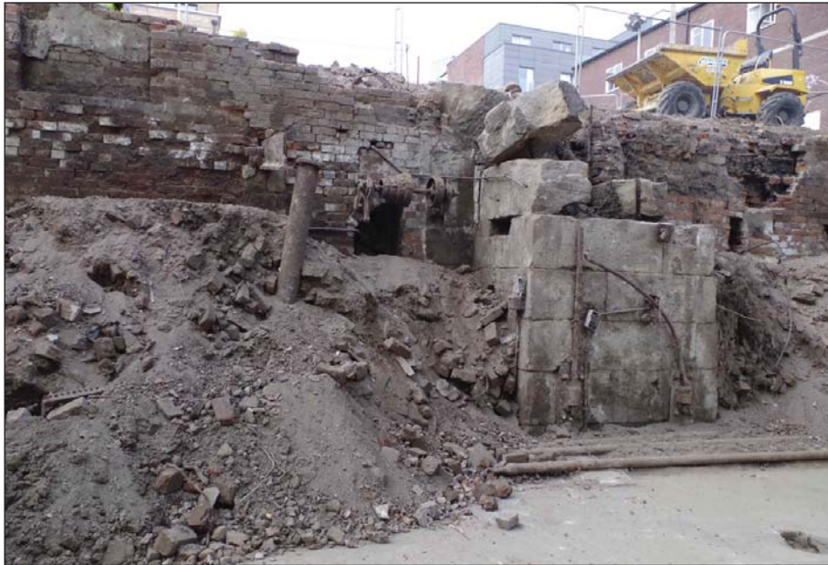
Plate 5: Oblique shot of middle part of main west wall 1013 from south-east
