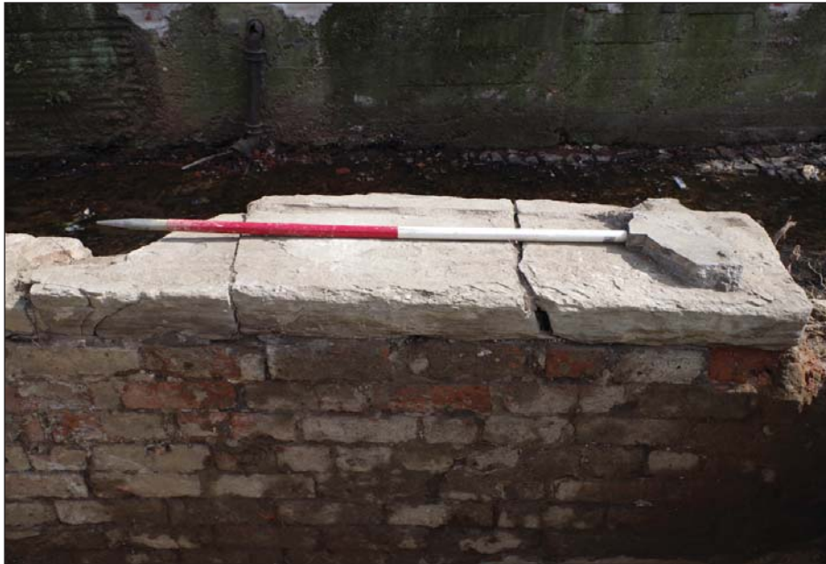
Plate 3: Window sill 1020 from west
