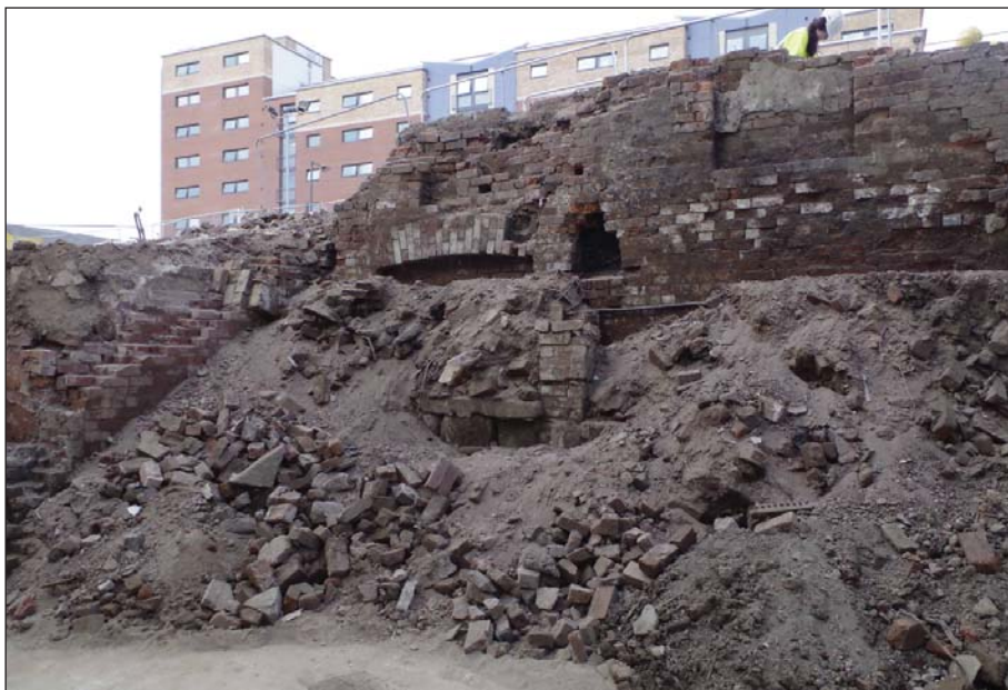
Plate 4: Oblique shot of south part of main west wall 1013 from north-east
