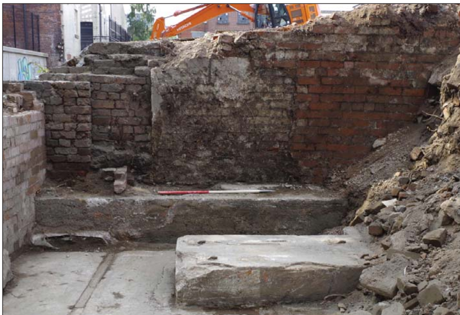
Plate 8: Southern wall 1023 of southern cellar from north
