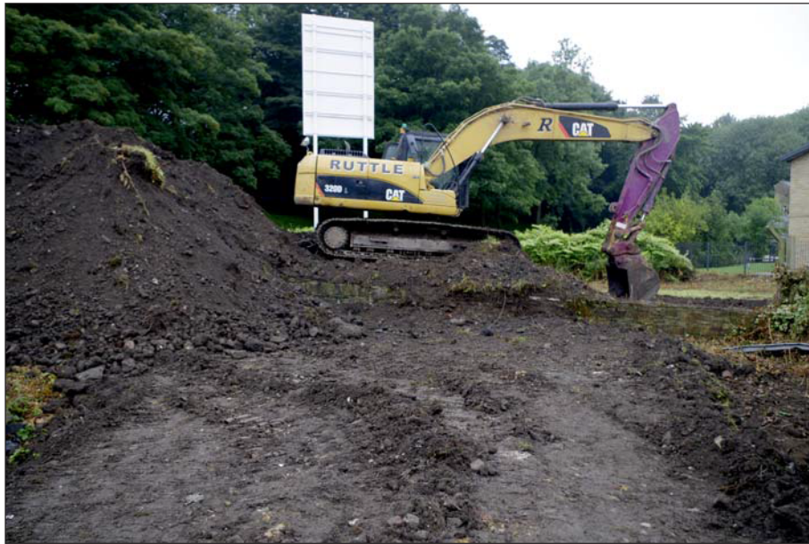
Plate 1: General shot of topsoil strip at southern limit of Site
