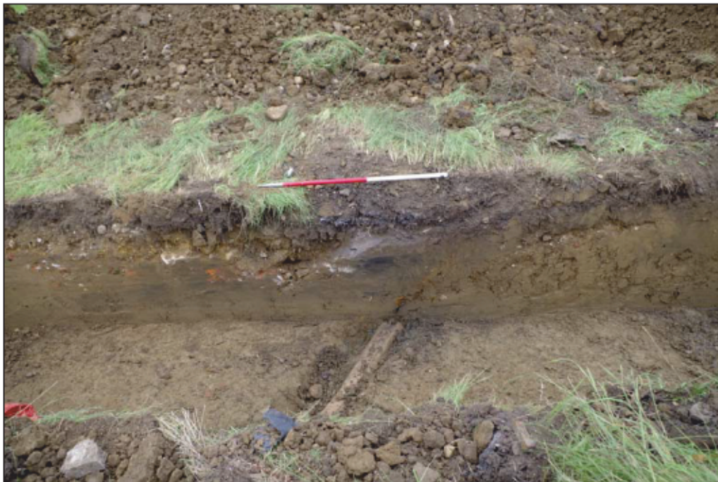
Plate 4: Cut containing modern land drain and associated fill, as seen in Trench 4
