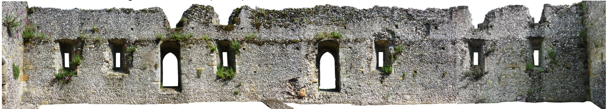
The brewhouse/bakehouse range's east wall, west (internal) elevation.
