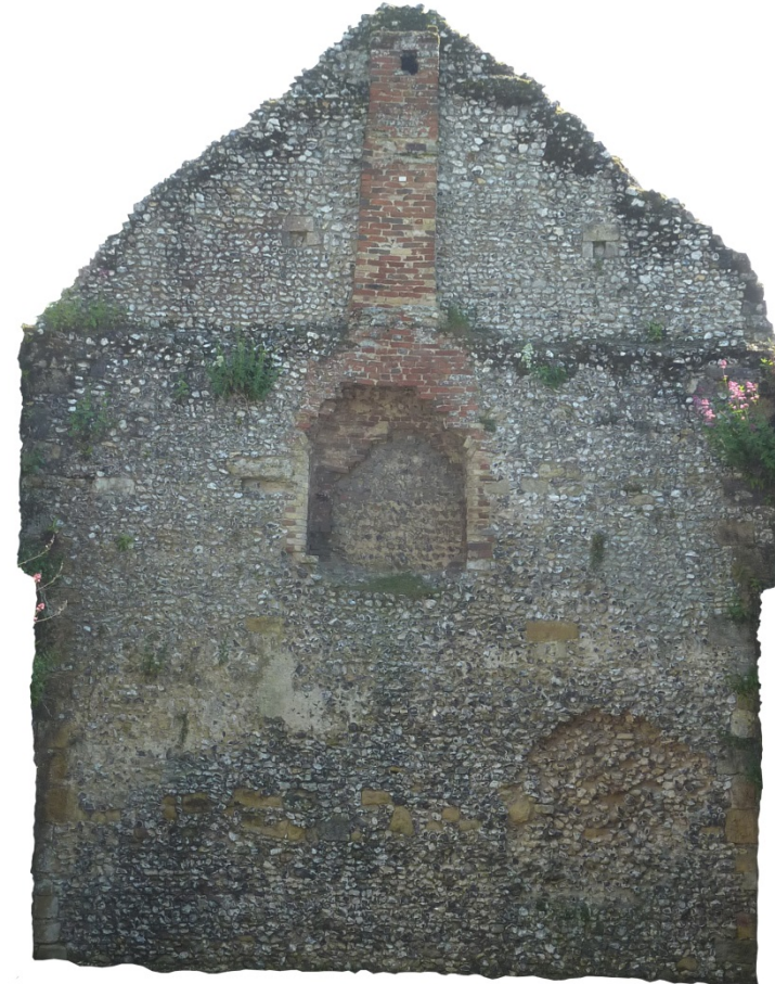
The brewhouse/bakehouse range's south wall, north (internal) elevation.
