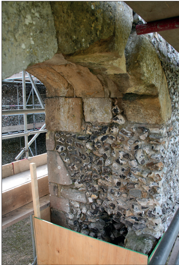
Plate 4: The head of the southwest entrance of the west wall showing broken masonry
