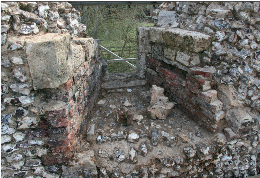
Plate 12: View from the west of a second floor window of the east wall with fragmented brickwork prior to its reinstatement
