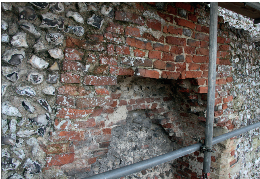
Plate 2: View of the brick fireplace on the northern elevation of the south wall
