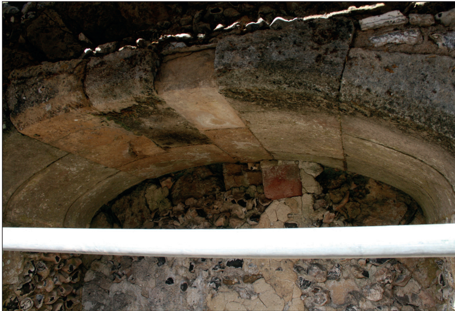
Plate 5: The head of the northwest entrance of the west wall showing replaced masonry
