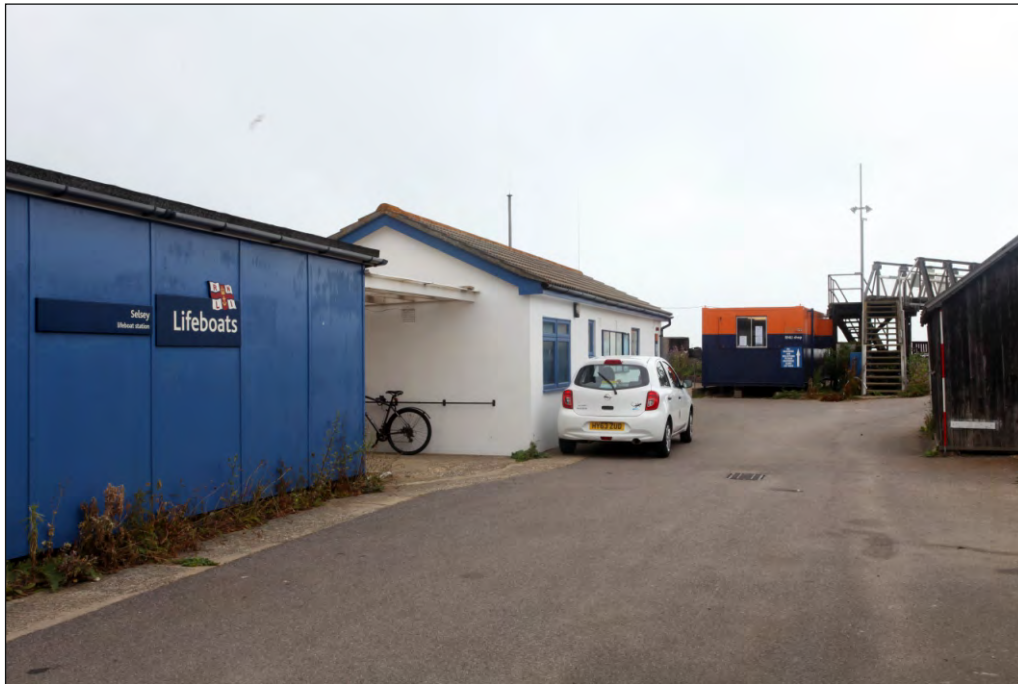
Plate 1: General view from the north-west of the onshore RNLI facilities.
