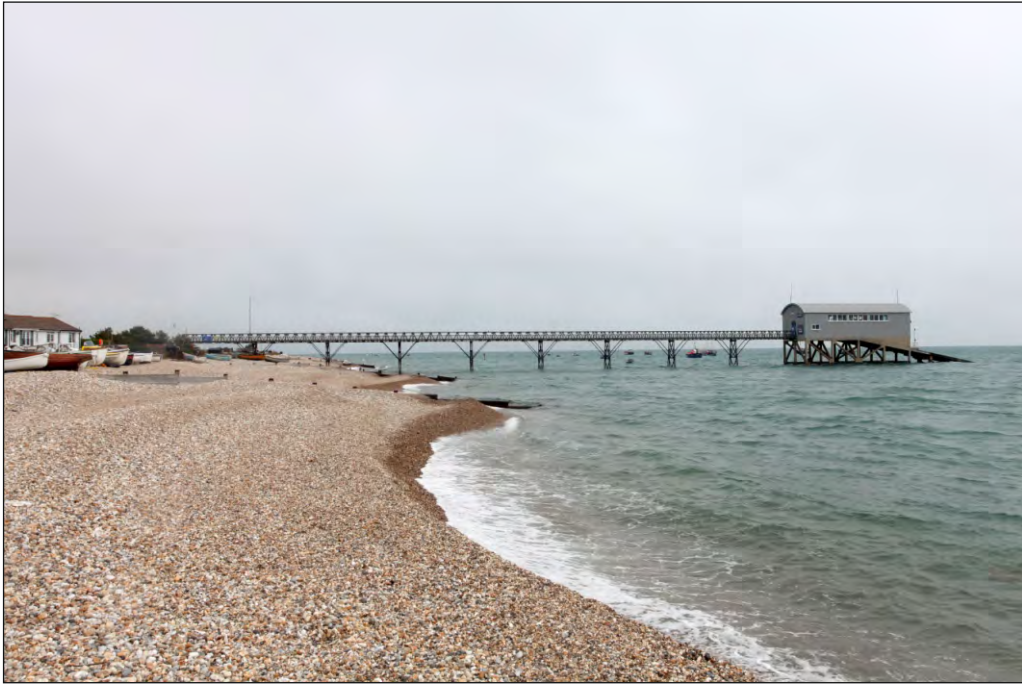
Plate 5: South-west elevation of the RNLI Lifeboat Station and the elevated walkway.
