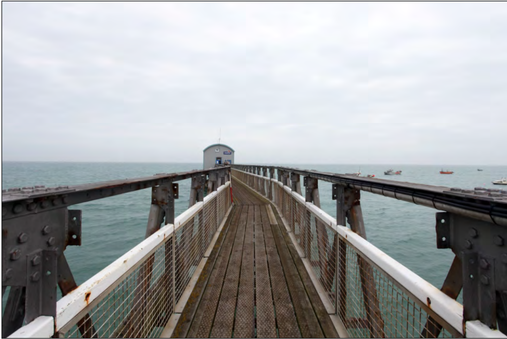
Plate 3: View from the north-west along the elevated walkway.
