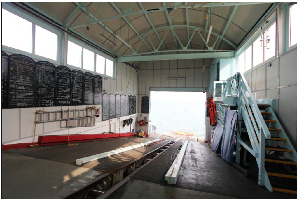
Plate 20: View from the north-west of the sloping boat ramp.
