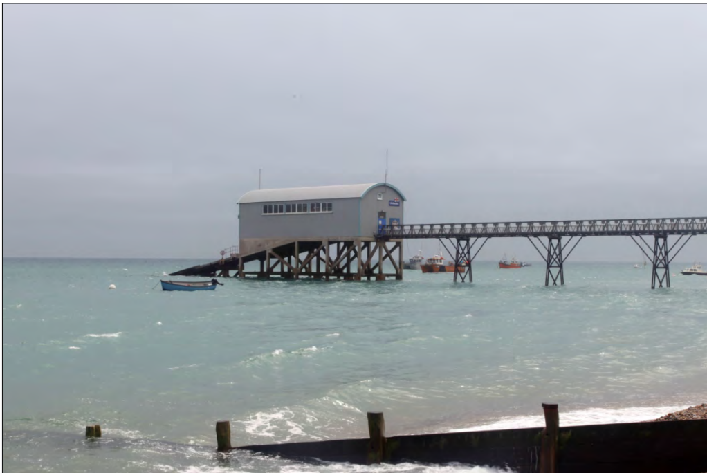
Plate 8: Oblique view from the north of the north-west and north-east elevations.
