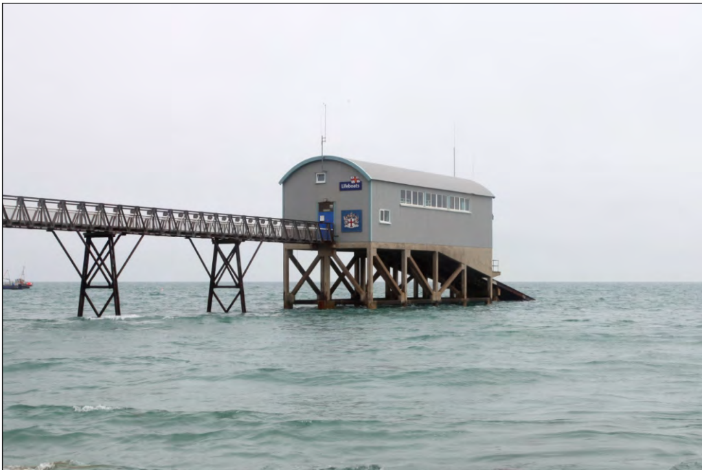
Plate 6: Oblique view from the west of the north-west and south-west elevations.
