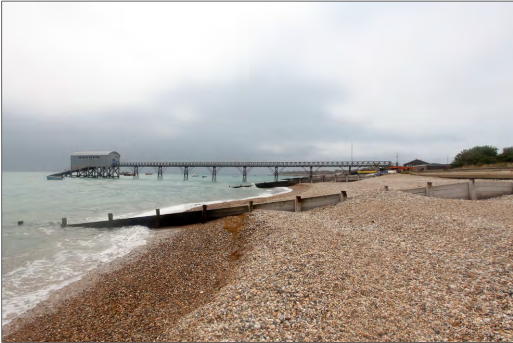
Plate 7: North-east elevation of the RNLI Lifeboat Station and the elevated walkway.
