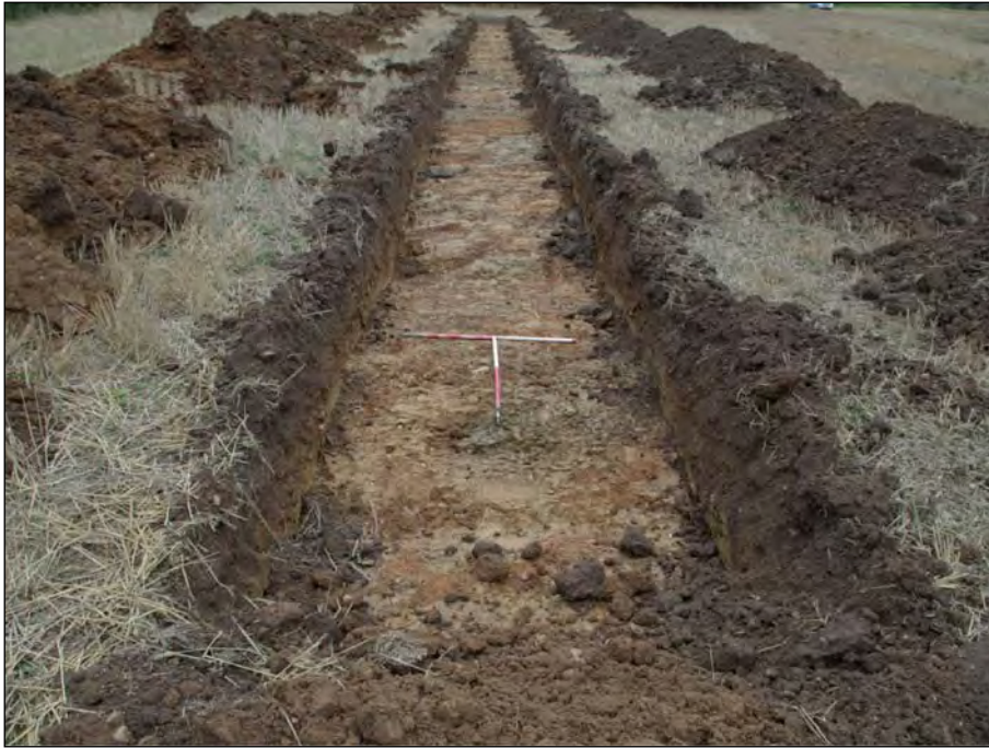
Plate 1: General shot of mottled natural geology, Trench 17
