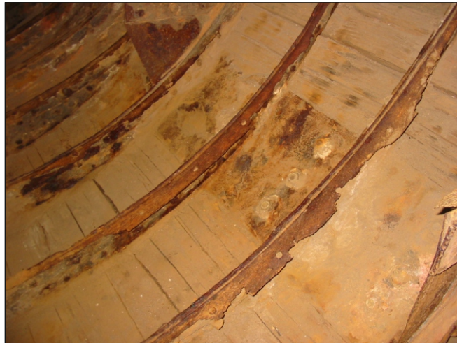
Plate 7: Interior of the hull, showing wooden planking and metal frames (2005)
