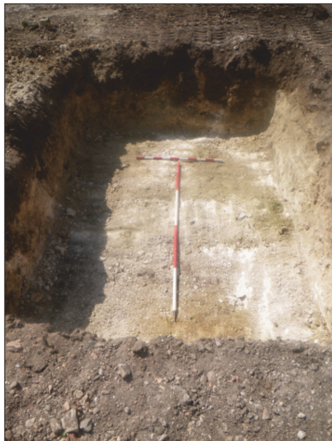
Plate 4: Excavated soakaway pit
