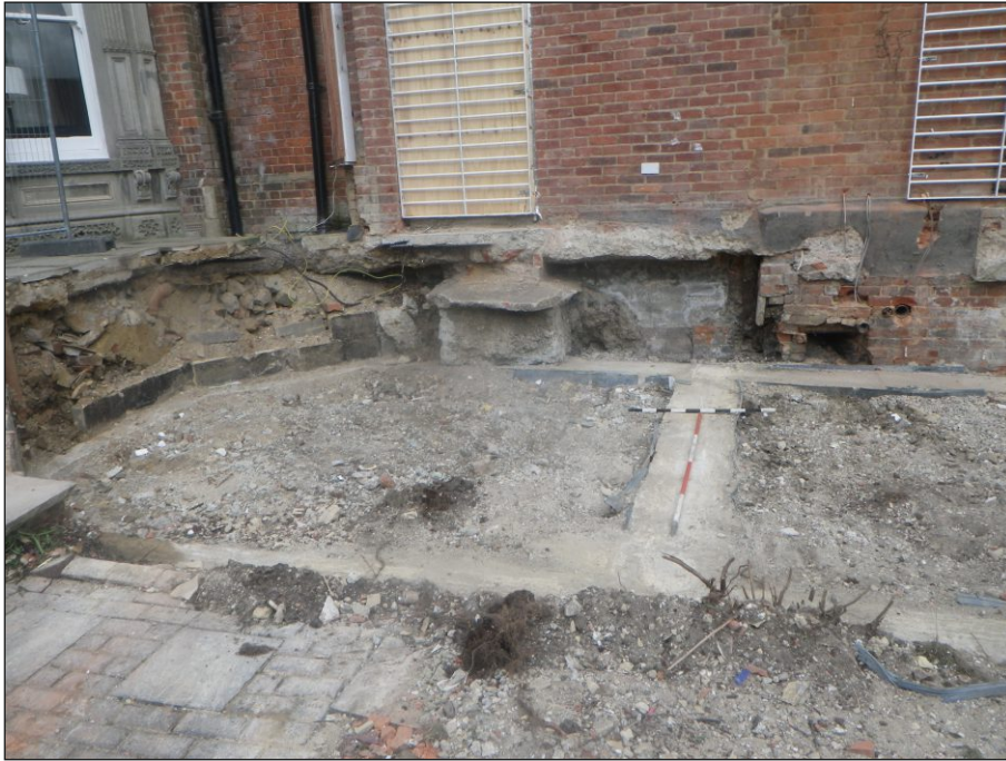
Plate 5: Area 6, view from the south-west
