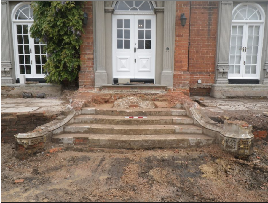
Plate 9: Entrance steps 710, view from the south-west
