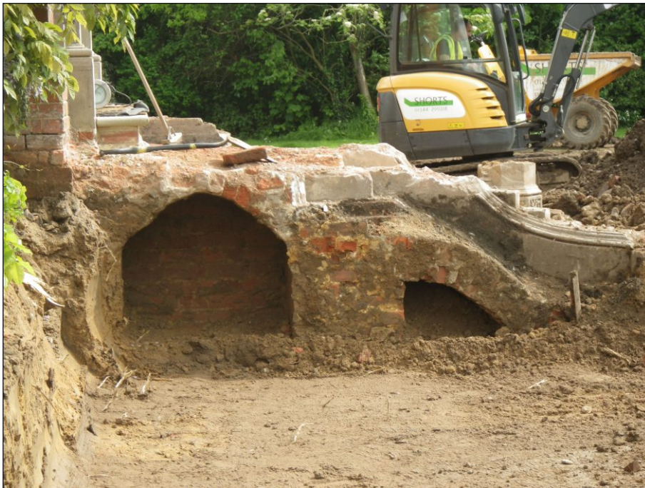
Plate 10: Brick support arches 708, view from the north
