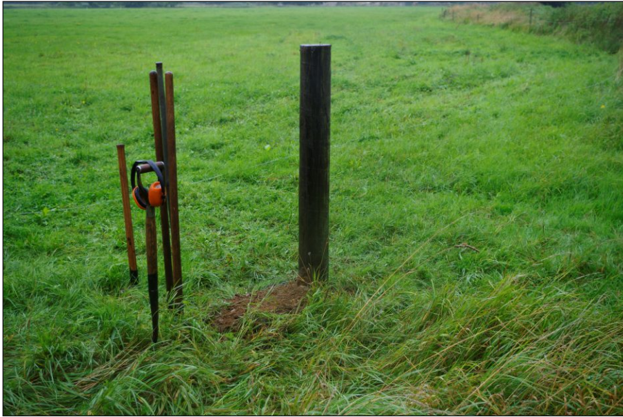
Plate 5: Replaced stock fence post
