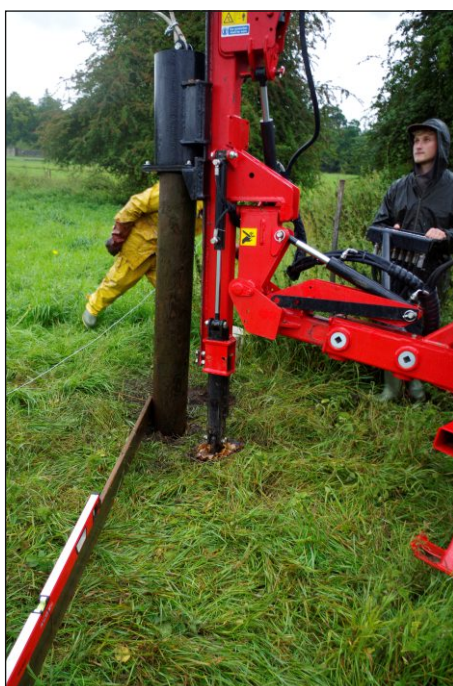
Plate 3: Replaced stock fence post
