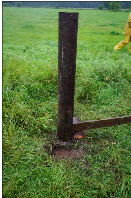
Plate 2: Replaced stock fence post
