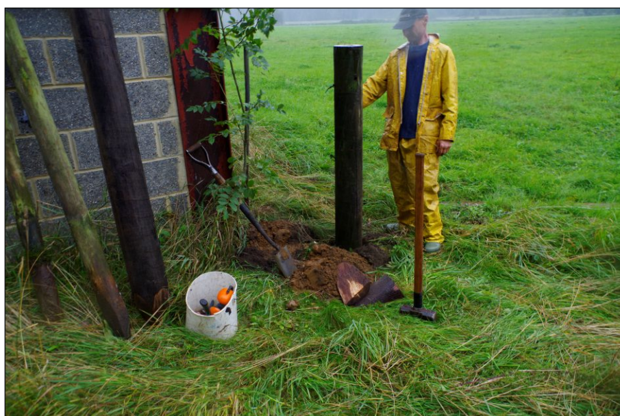
Plate 4: Replaced stock fence post
