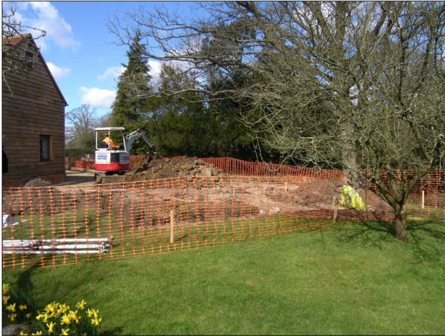
Plate 1: Shot of building footprint being excavated, view from the south
