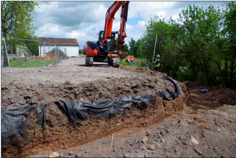
Plate 3: Excavation of sheet pile guide trench to the west of Willow Tree Cottage, looking north-east
