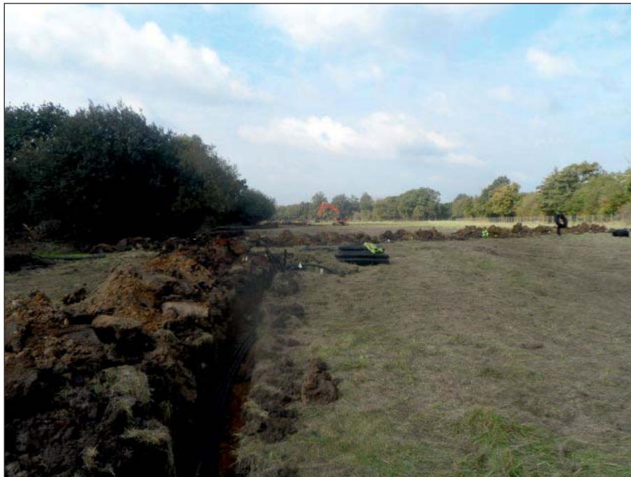
Plate 6: Main electrical cable trench through northern field, viewed from the south-east
