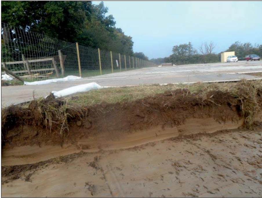
Plate 1: South-east facing section access road adjacent to new bridge
