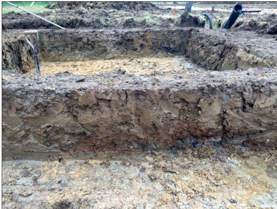
Plate 9: East facing section foundation trench for inverter cabin
