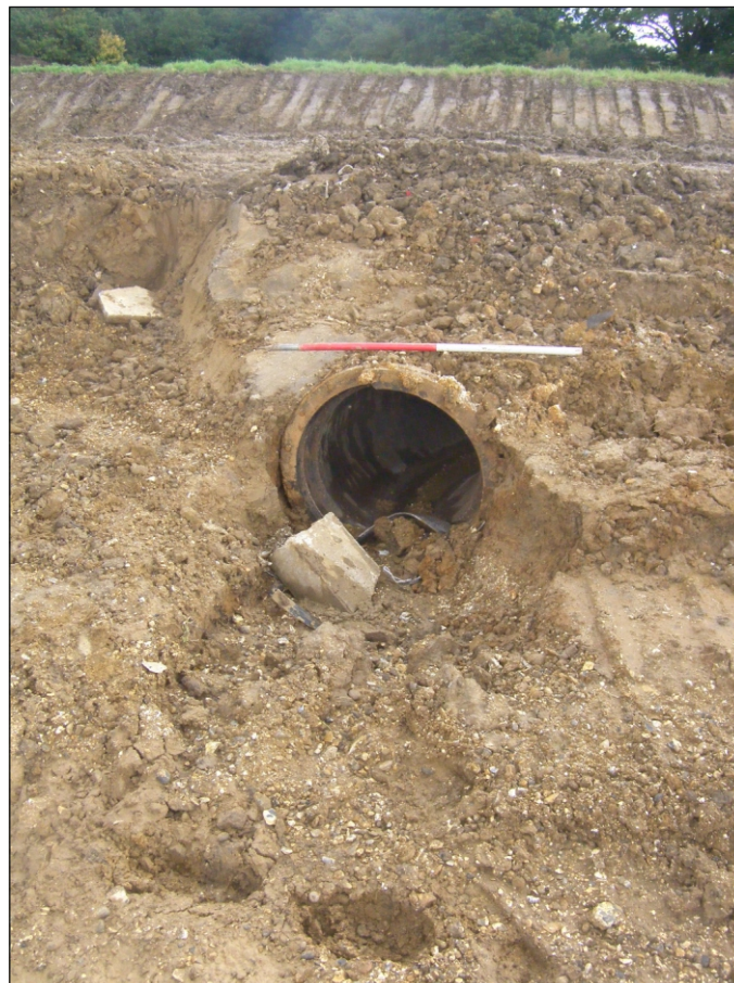
Plate 4: Modern concrete drain 1021 on the east side of Site, viewed from the west.
