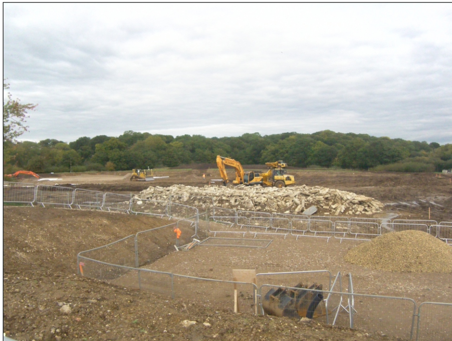
Plate 2: View of the Site from the west showing the concrete spoil from a modern drainage channel demolished prior to the watching brief.
