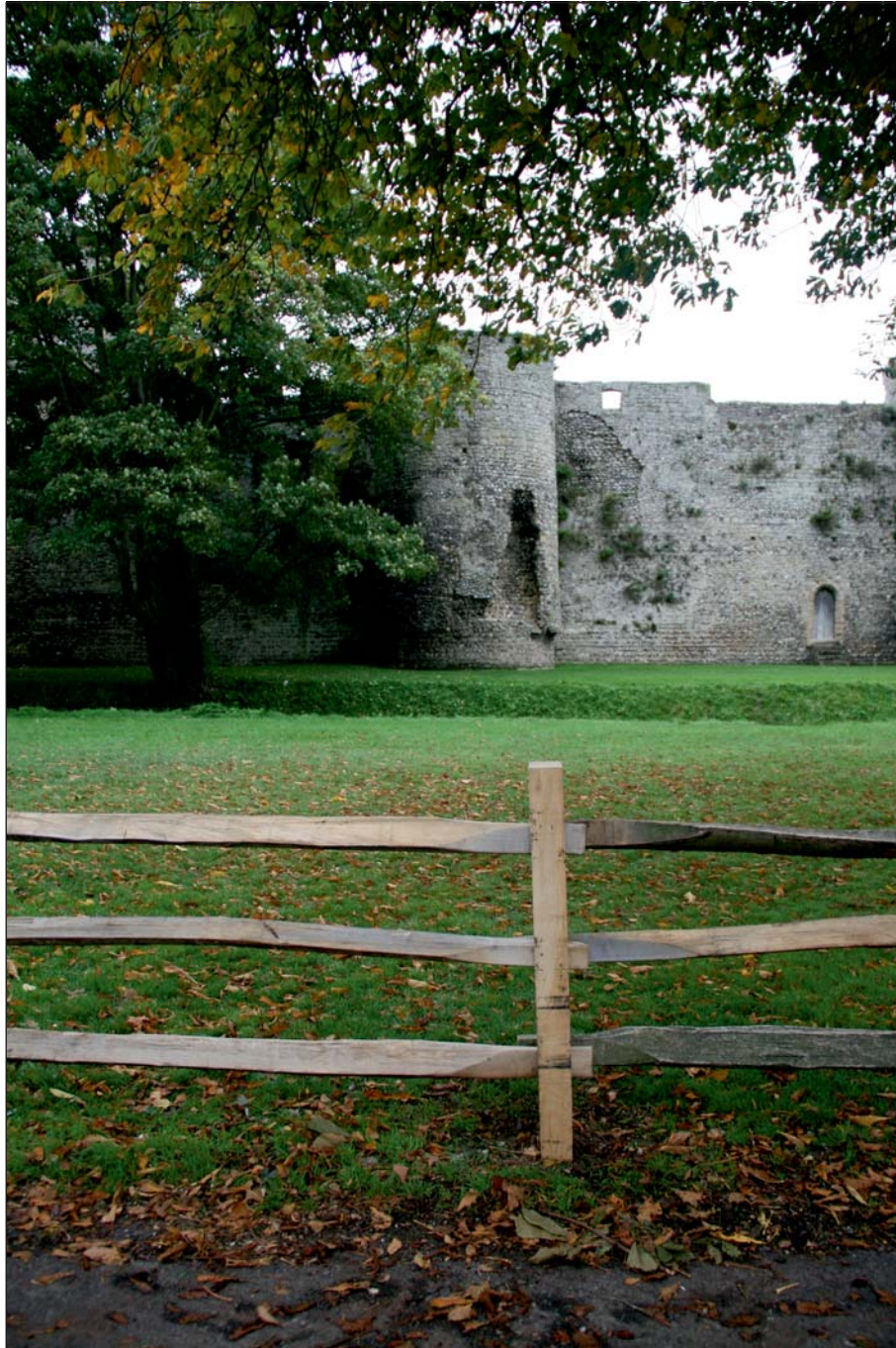
Plate 3: The repaired fence with installed replacement post and staves, looking south
