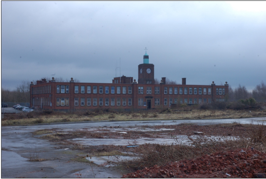
Plate 1: Clocktower Building from the west
