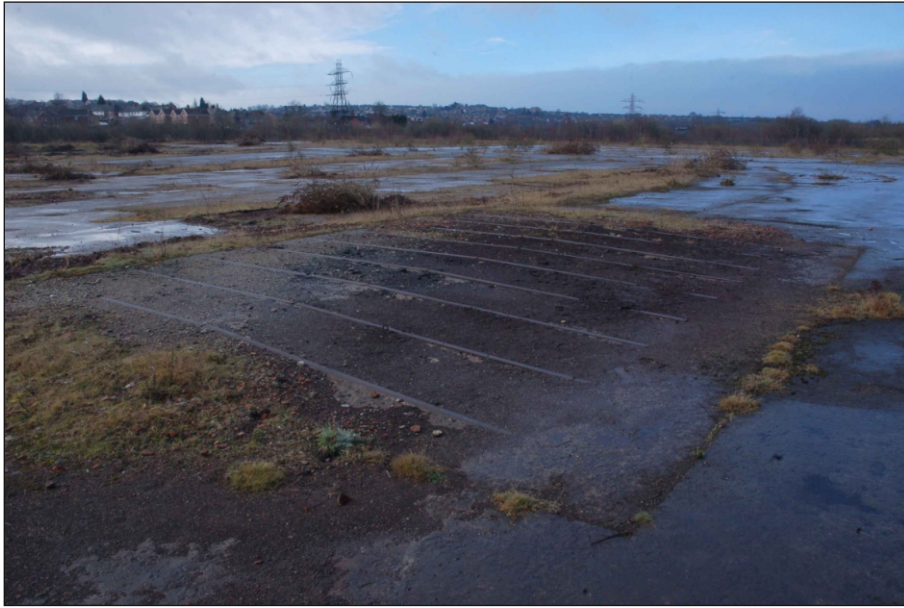
Plate 9: Railway lines visible within the Site
