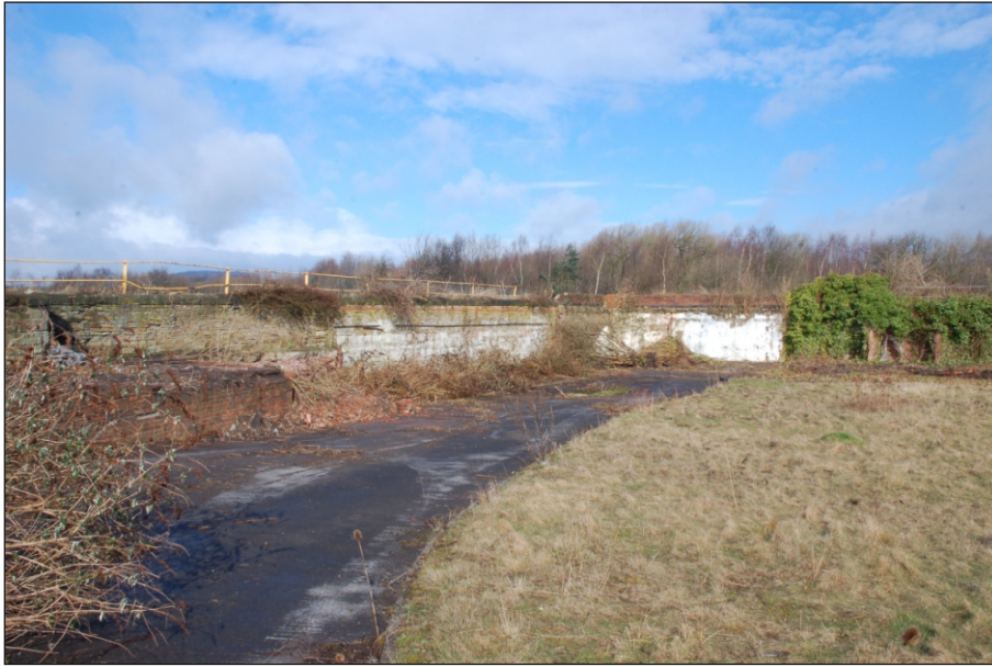
Plate 5: Walls from former industrial buildings remaining on Site
