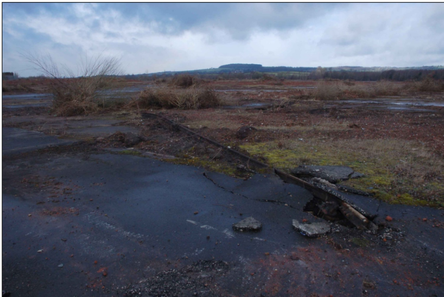
Plate 10: Railway lines visible beneath hardstanding
