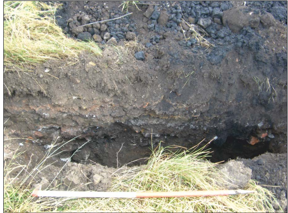
Plate 2: TP216 looking west
