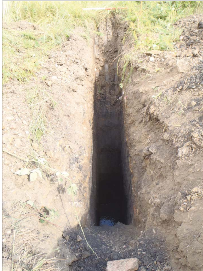
Plate 7: TP232 looking south
