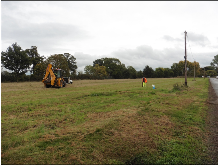
Plate 1: Northern edge of OA 2, camera facing south-east
