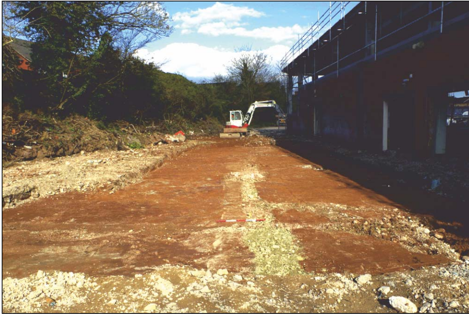
Plate 1: General view of Trench 1 from the south-west
