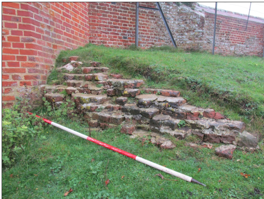
Plate 8: Brickwork visible at turret base, view from the south-west
