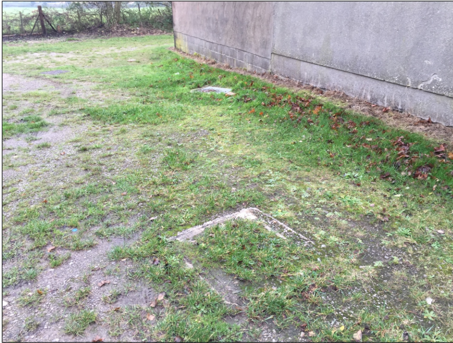
Plate 5: Man hole covers over septic tanks in Field 3 behind Sports Hall
