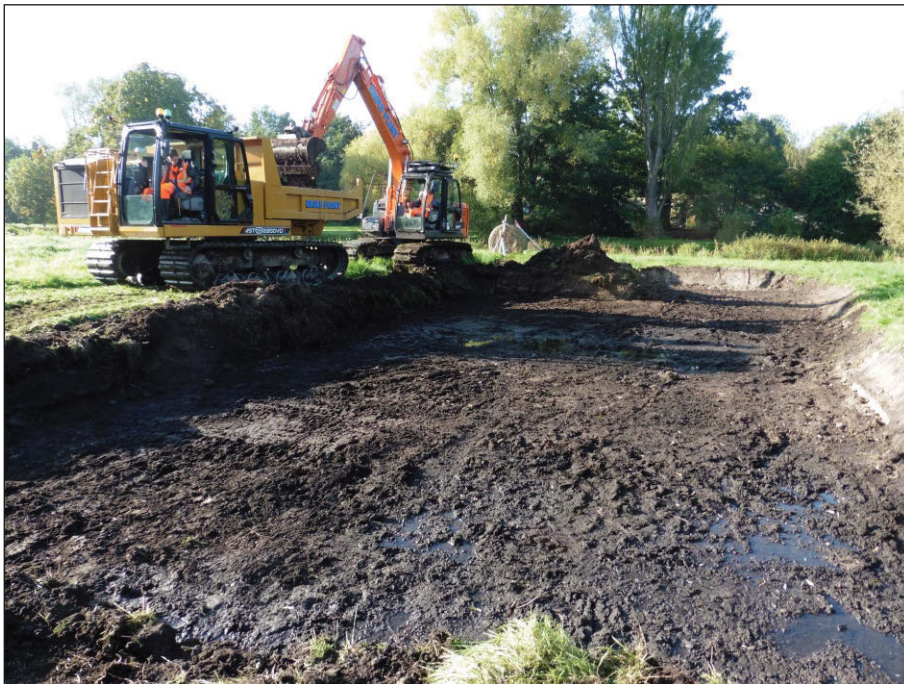
Plate 2: Mechanical excavation of Shallow Scrape
