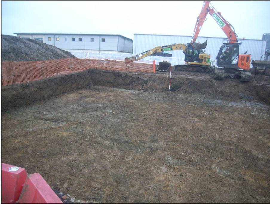
Plate 1: General shot of site stripping
