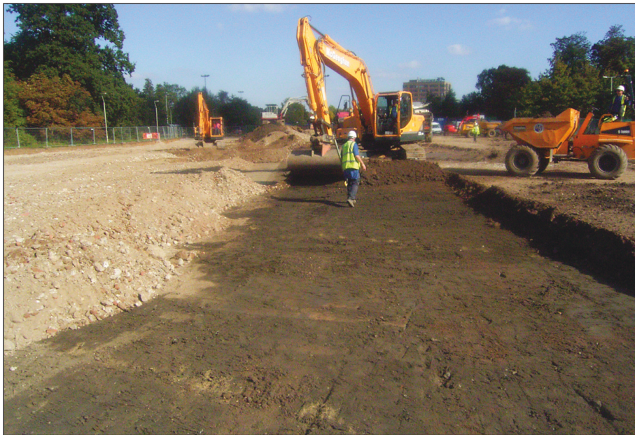
Plate 4: Machining surface of dark silty clay within palaeochannel: also showing laying of aggregate for car park base.
