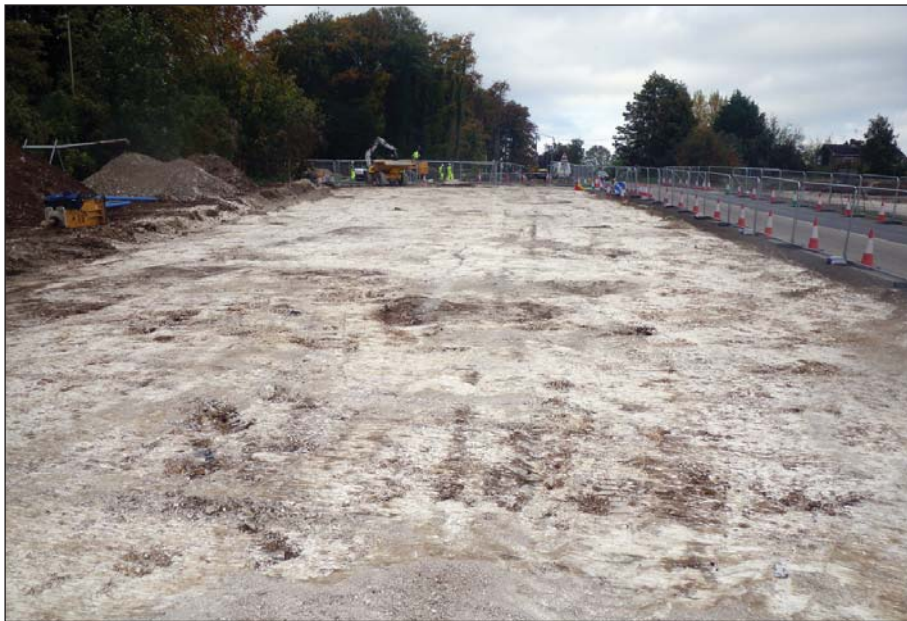
Plate 2: North-west facing shot of stripped Area 1
